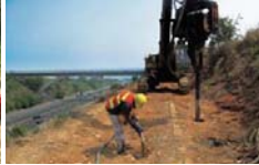
邊坡補強 | Slope Reinforcement
