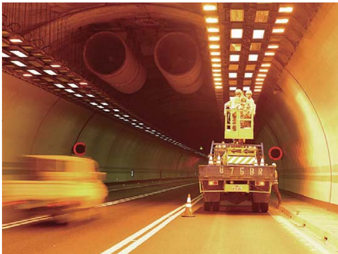
隧道燈具維護 | Maintenance of Tunnel Lighting
