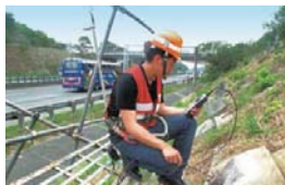
地錨檢測 | Ground Anchor Inspection
