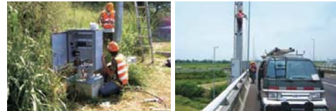
路側式車輛偵測器安裝 | Installation of A Roadside Vehicle Detector
