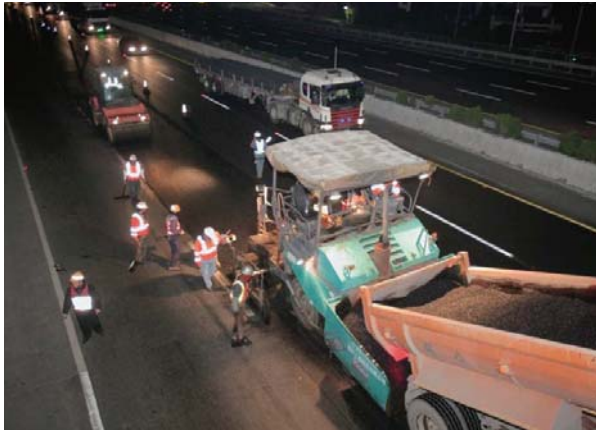
夜間道路救援 | Nighttime Road Work
