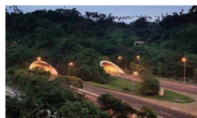
高雄3號國道隧道 (夜) | Lantian Tunnel, National Freeway No.3 (At Night)
