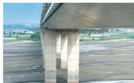
橋梁檢測 | Bridge Inspection
