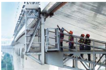
橋梁檢測 | Bridge Inspection
