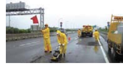
抗壓緊急維修 | Emergency Pothole Repair
