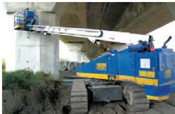
橋梁檢測 | Bridge Inspection
