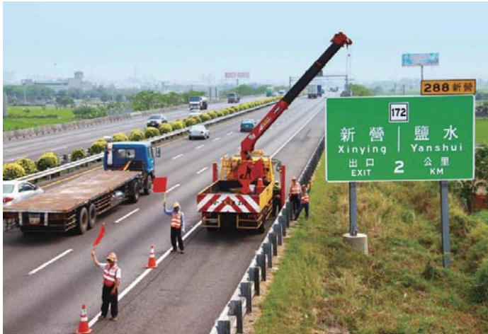
標誌施工 | Traffic Sign Construction
