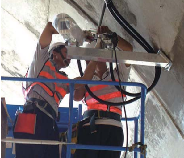
事件自動偵測系統安裝 | Installation of An Automatic Incident Detection System
