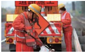
碎渣物清除 | Debris and Litter Removal
