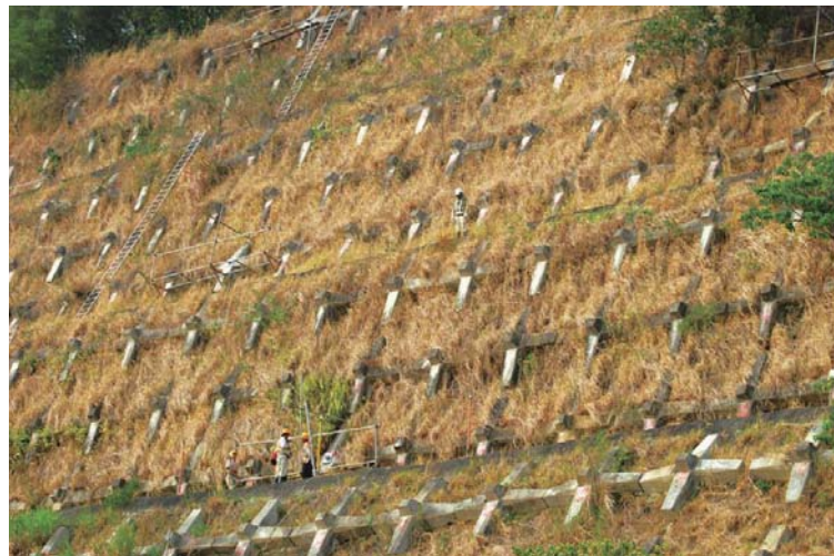
地錨檢測 | Ground Anchor Inspection
