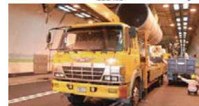
隧道風扇安裝作業 | Installation of Tunnel Ventilation Fan
