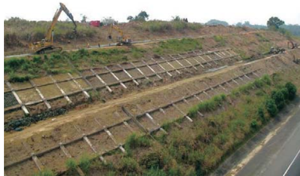
邊坡補強 | Slope Maintenance
