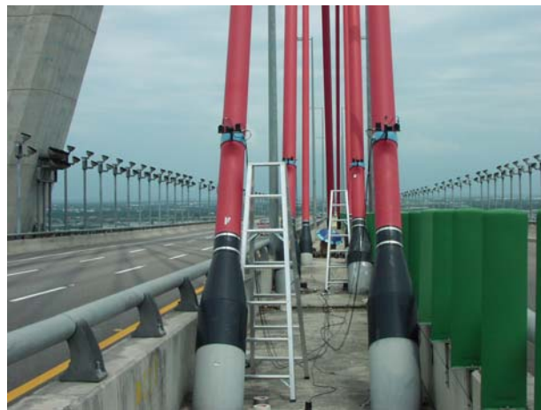
Figure 2.3 Arrangement of Stay Cables in Pairs
