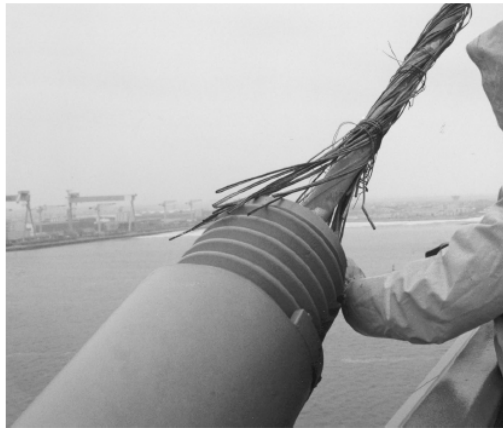
Figure 1.1 Rupture of stay cable due to fatigue (Siegert and Brevet 2006)
