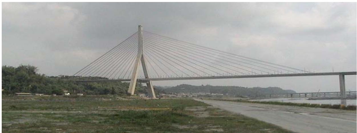
Figure 2.1 The Kao Ping Hsi Cable-Stayed Bridge
