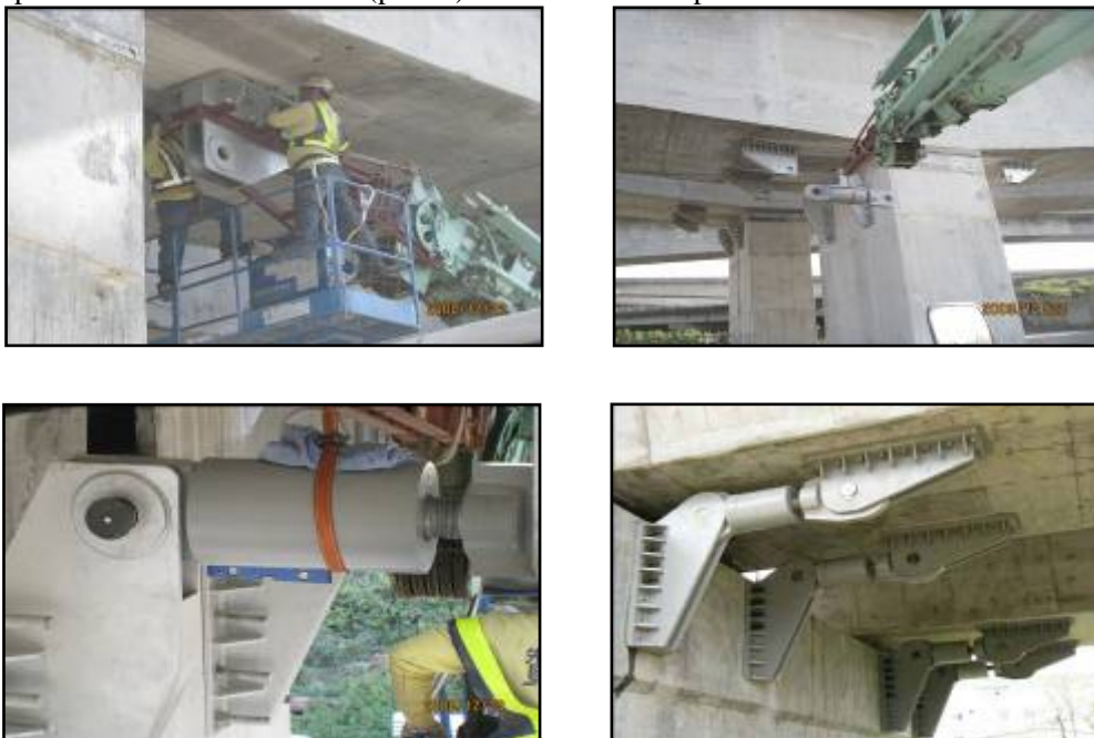
Figure 19 STU Installation Work
