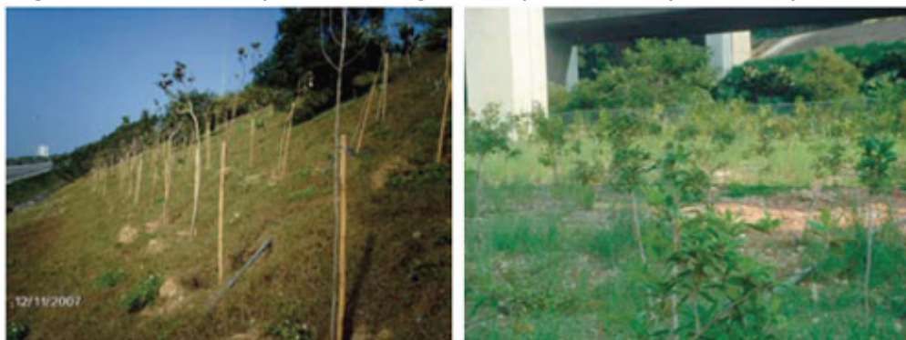
Ecological vegetation at Chunan Interchange and Dajia Interchange
