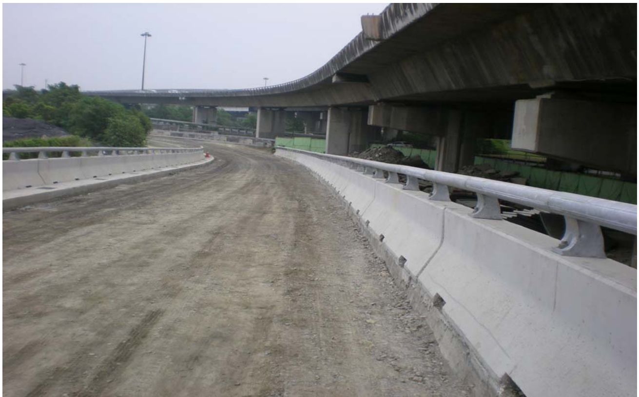
Ramp construction works
