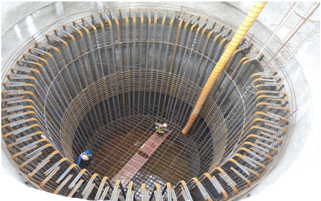
Dahua System Interchange Project – EP8 tube foundation structure's steel bar binding works
