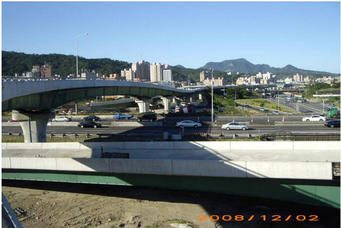
Project No. 204— Work on ramps A, B and C.
