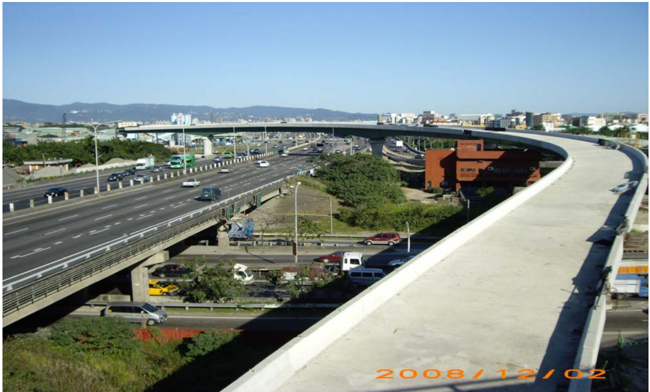
Project No. 204 — Work on Elevated Ramp C.
