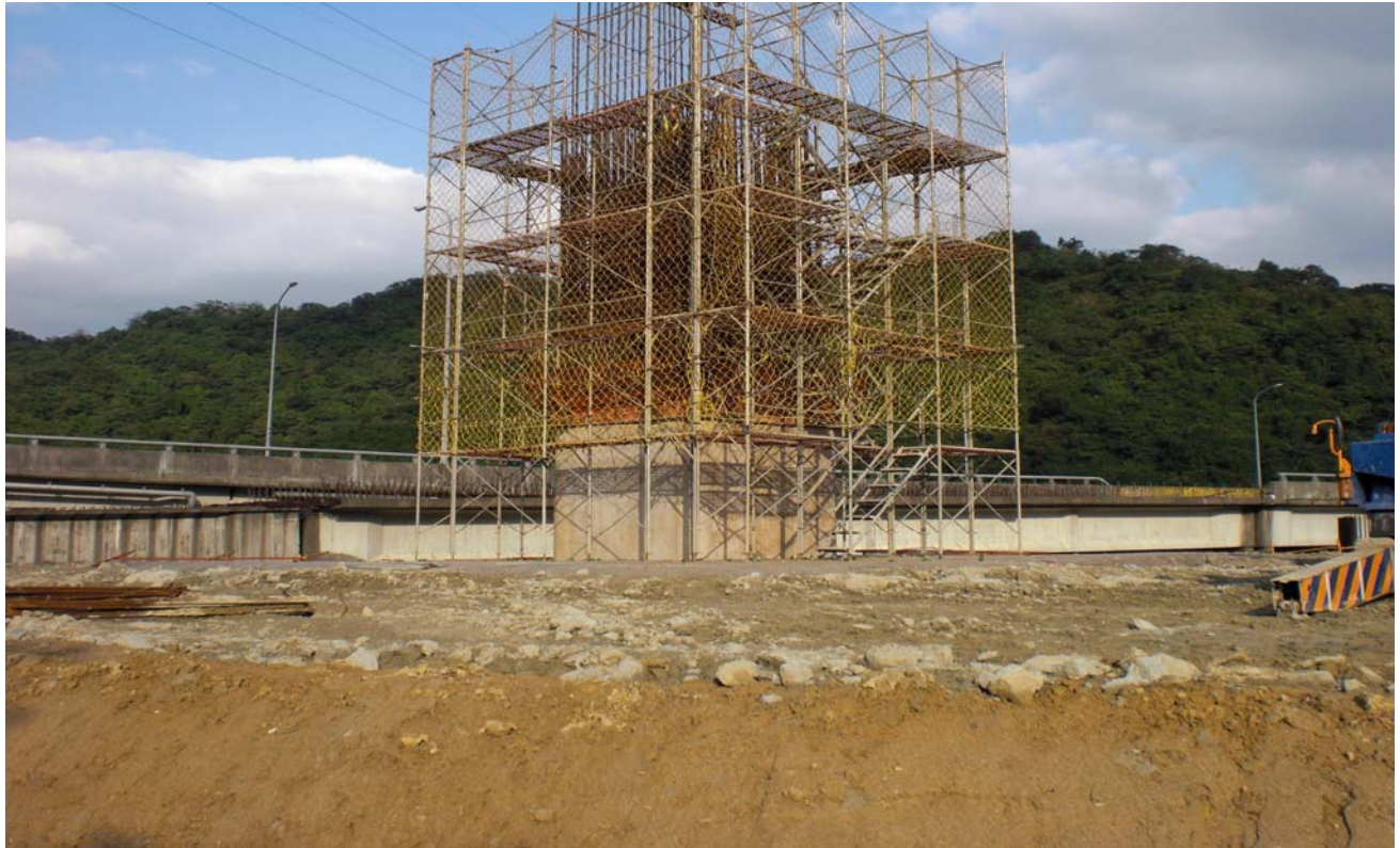
Dahua System Interchange Project – EP14 pier foundation steel bar binding works.
