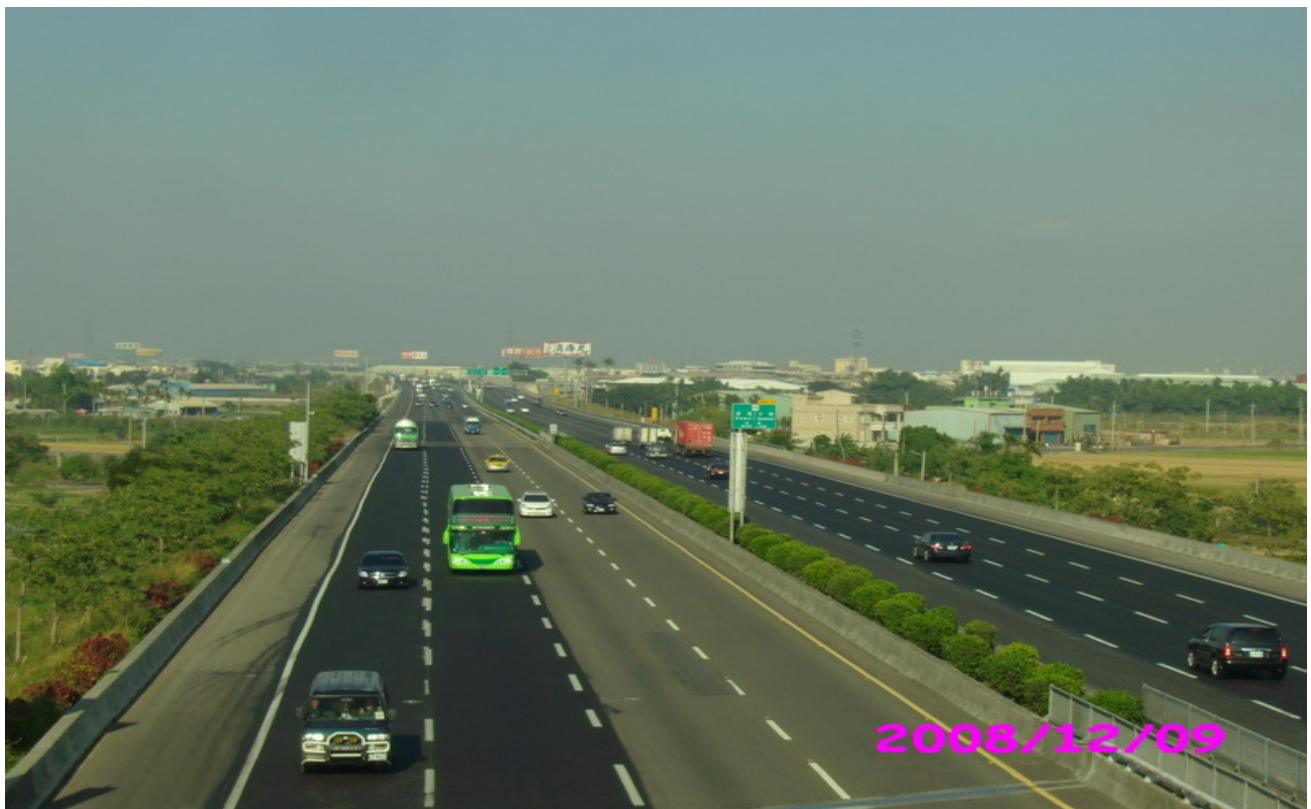
Project No. 521— 4 Lanes opened in June 15 th 2008
