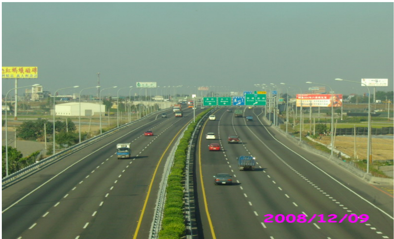
Project No. 521— 3 Lanes opened in June 15 th 2008
