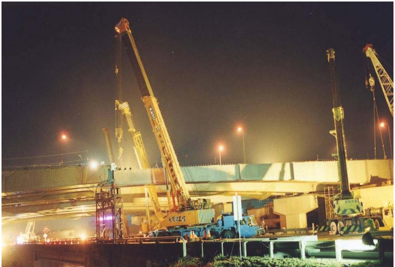
Closing of the National Freeways at night for setting up the beams
