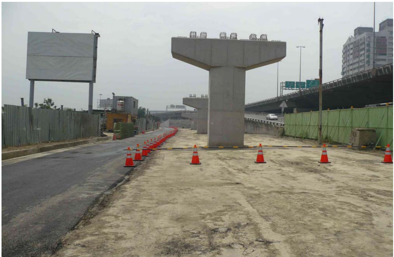
Bridge pier works completed
