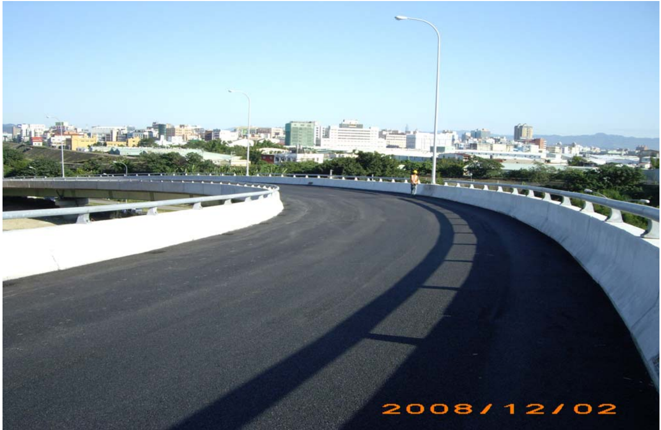
Contract No. 204— Ramp Bridge A roadwork
