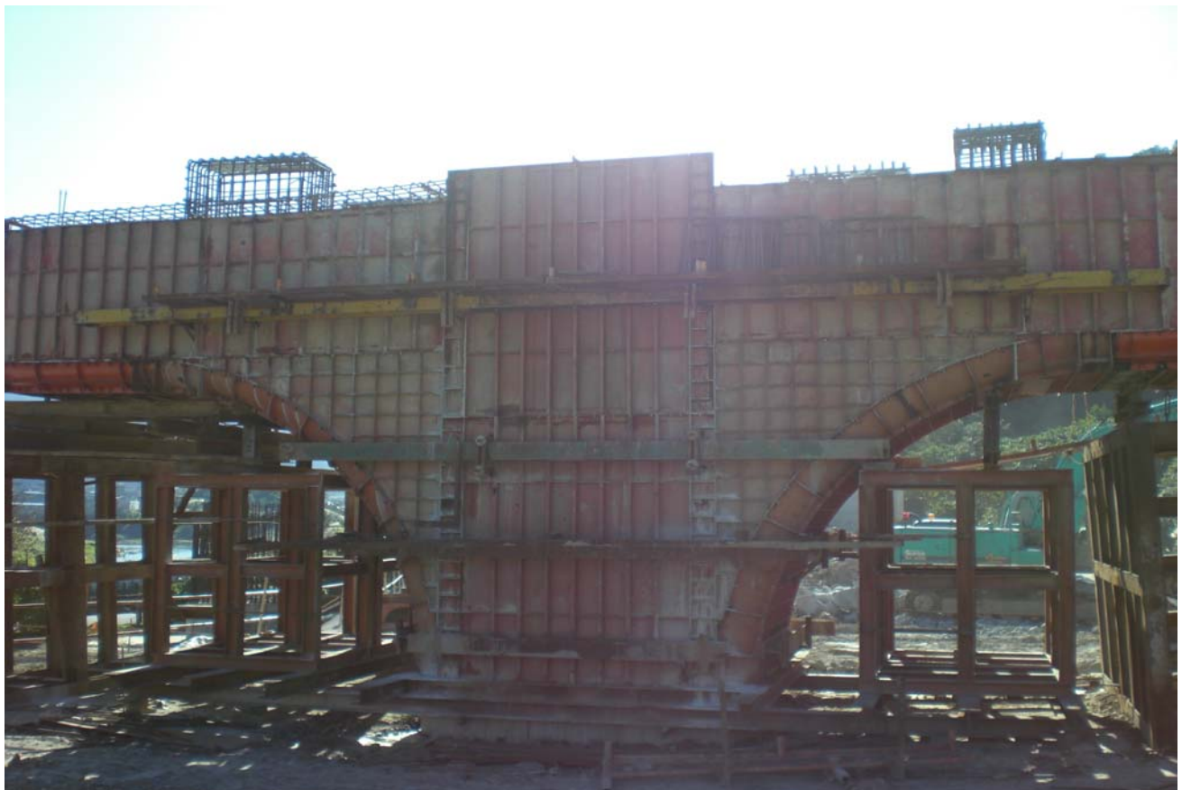
Dahua System Interchange Project – H2P6 beam construction.
