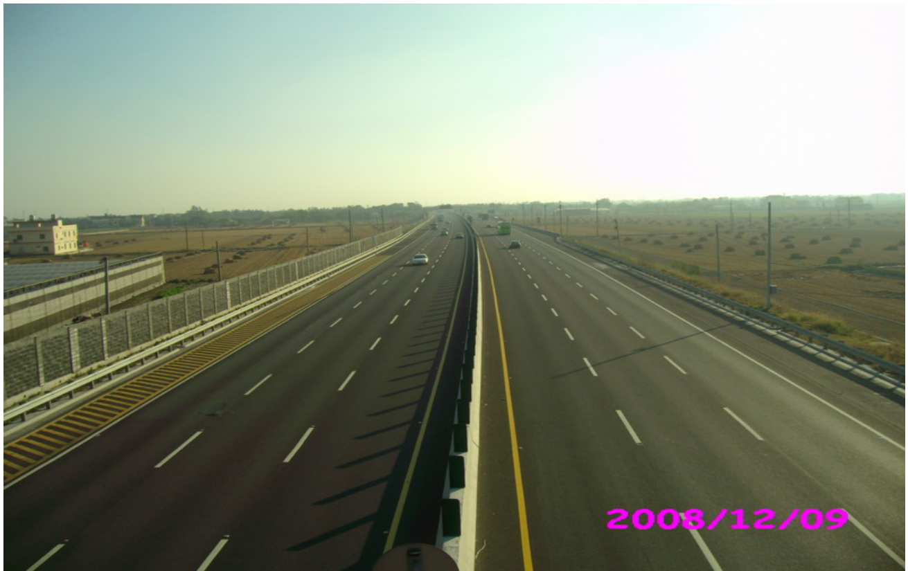
Project No. 521— 3 Lanes opened in June 15 th 2008
