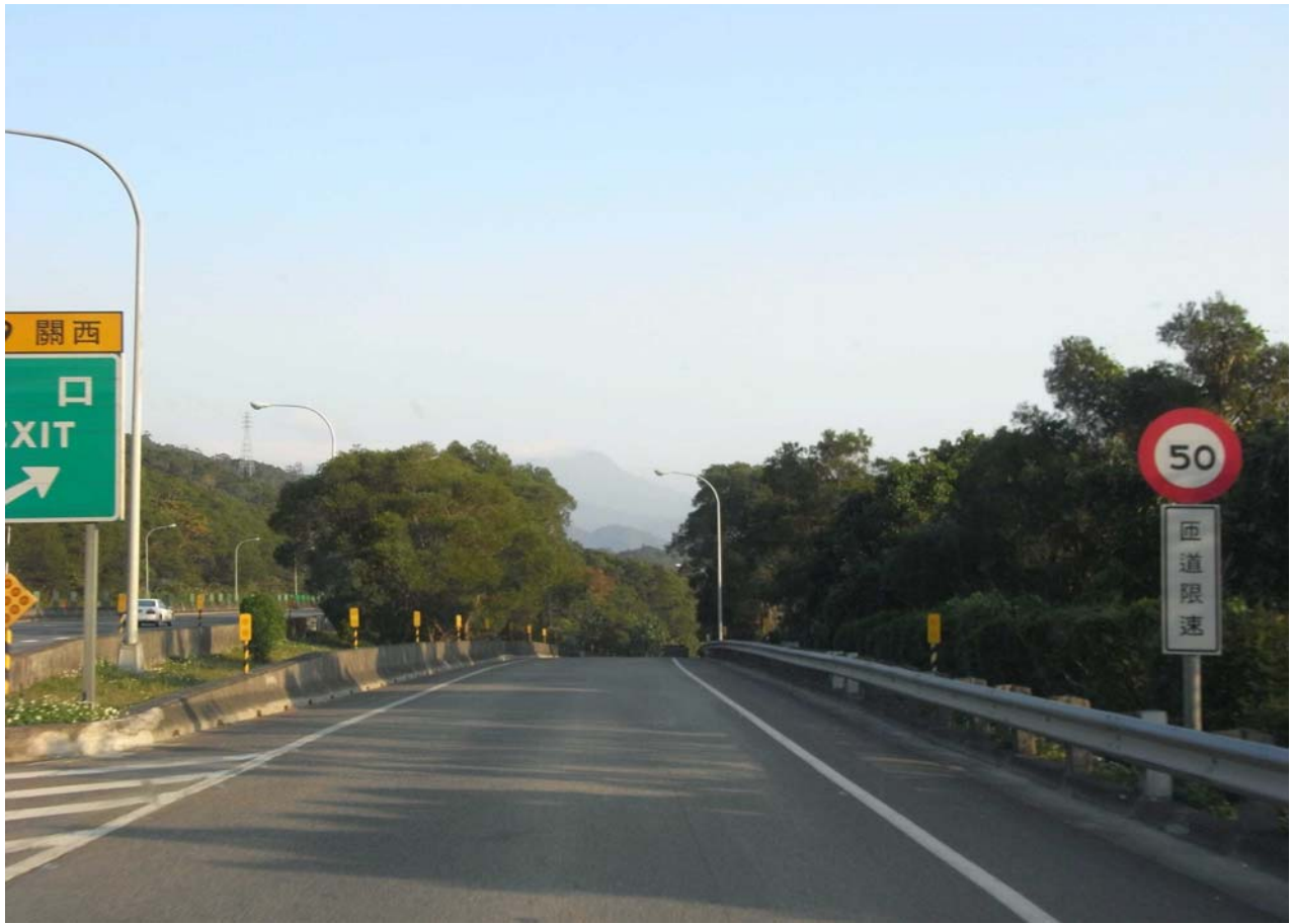
Guansi interchange ramp scenery
