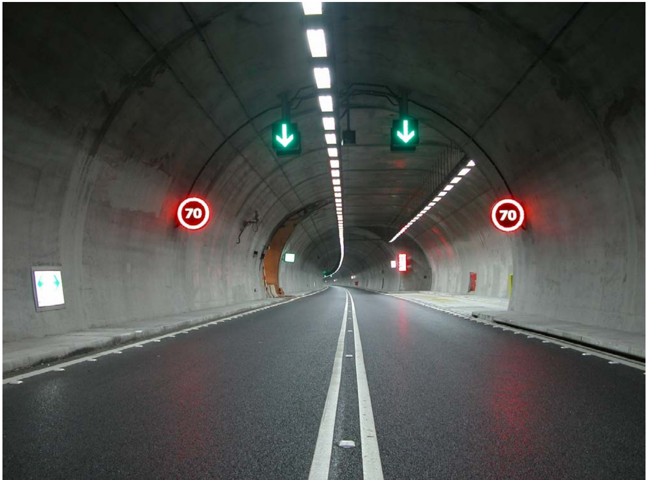
Freeway No.5 Hsuehshan tunnel
