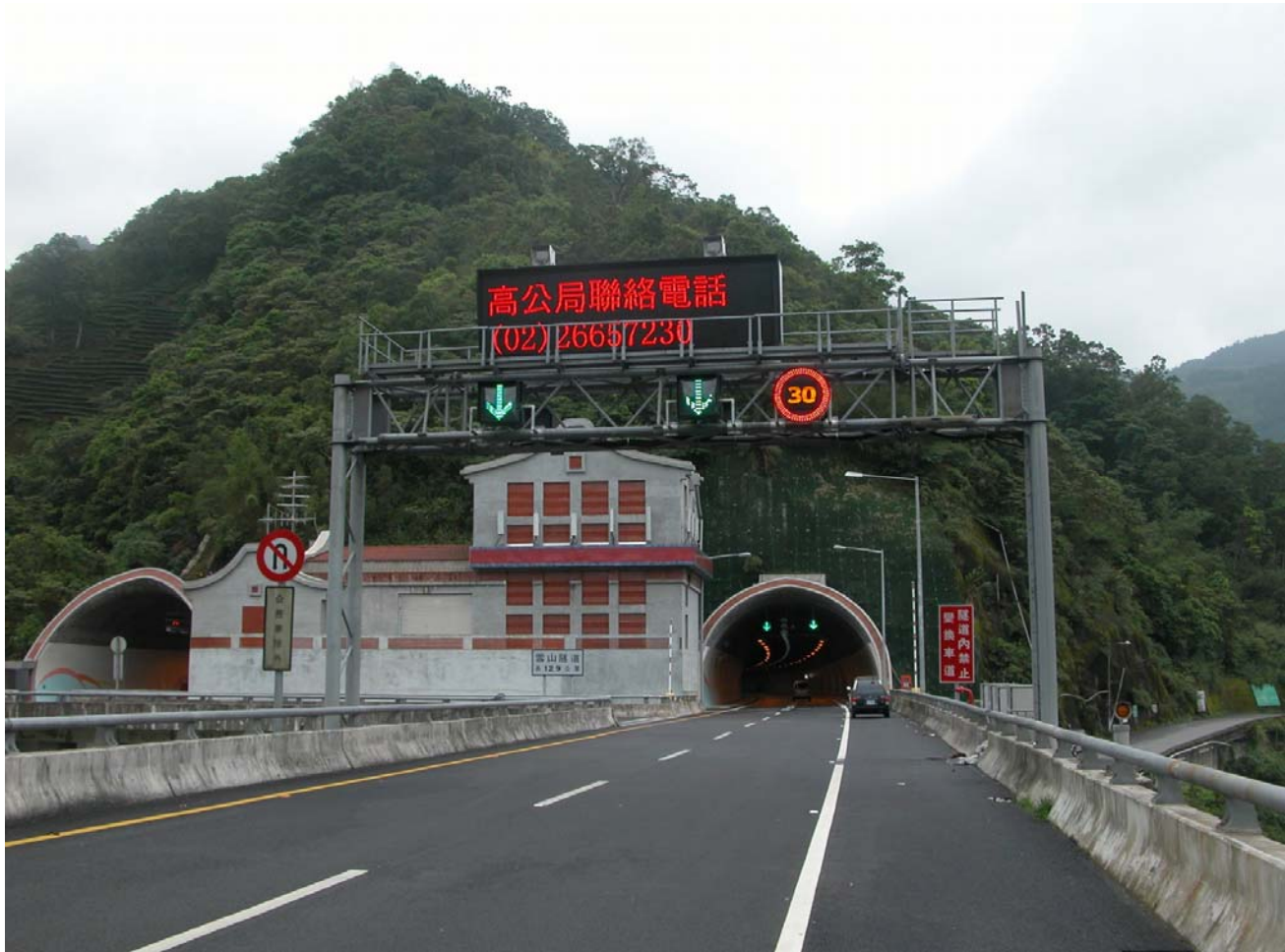
Freeway No.5 Hsuehshan tunnel north opening
