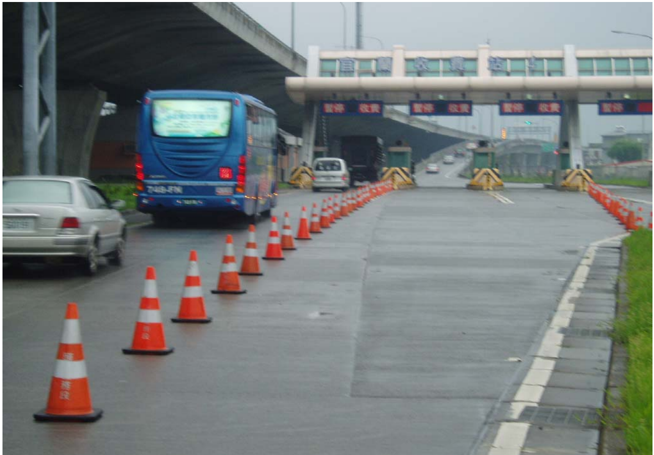
Yilan interchange entrance toll station traffic cone placement to improve traffic order.
