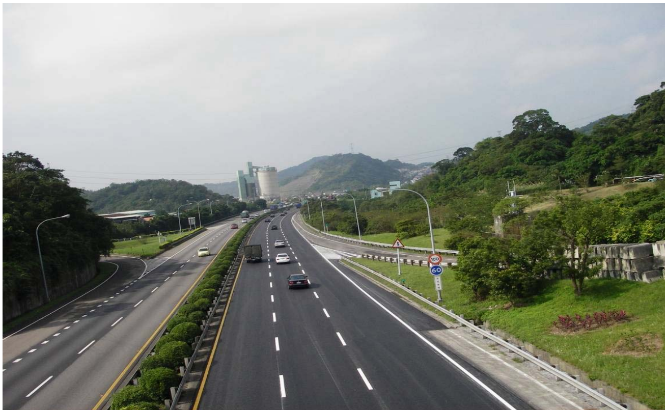
National Freeway No. 1 Wudu southern interchange section is widened to by auxiliary lanes to 3 lanes from 2.
