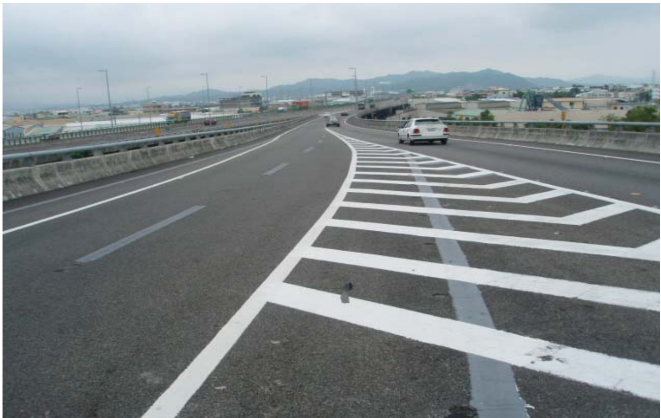
Adjustments to 2 laned access road of Southbound traffic exiting National Freeway No.1 to National Freeway No.4 (towards Dongshi). The 2 lanes are reduced to 1 lane traffic.
