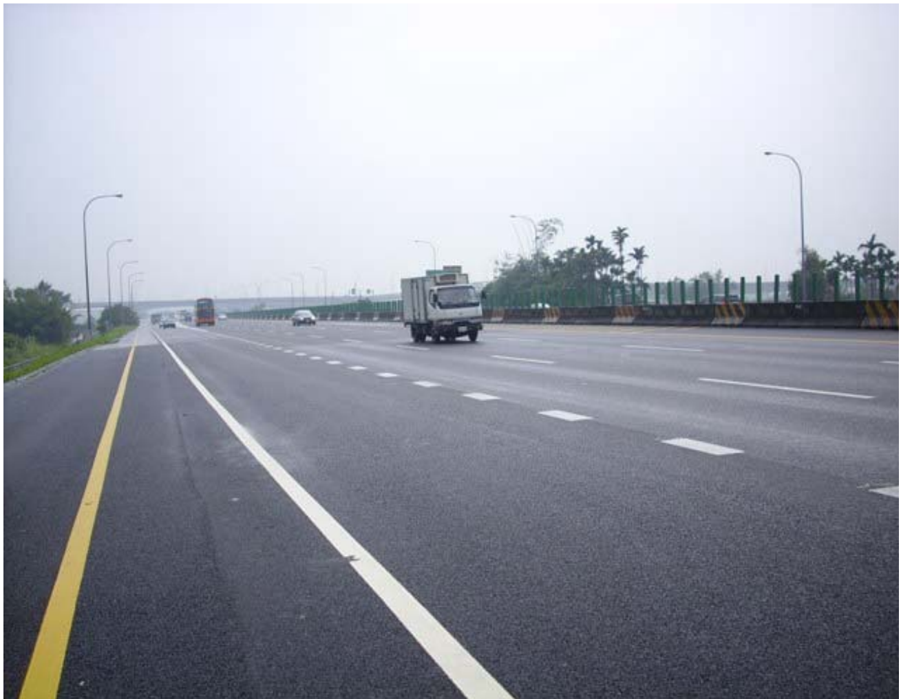
Photo of the extended access lane northbound entering National Freeway No. 1.
