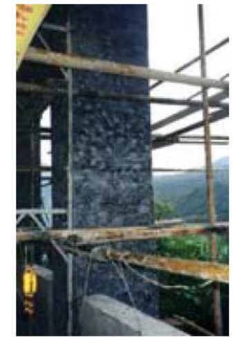
(a)Filling crack (b)FRP attachment (c)Placing cement
