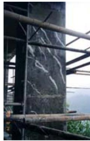
(a)Filling crack (b)FRP attachment (c)Placing cement
