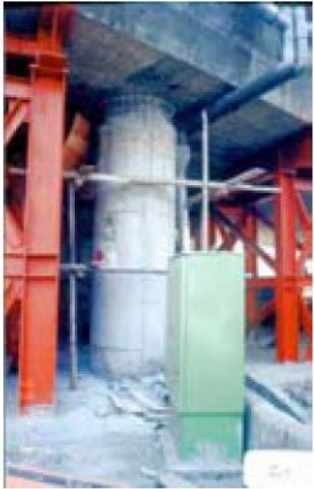
(a)Knocking RC (b)Section recovery (c)Surface grind
