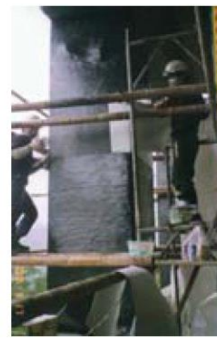
(a)Filling crack (b)FRP attachment (c)Placing cement
