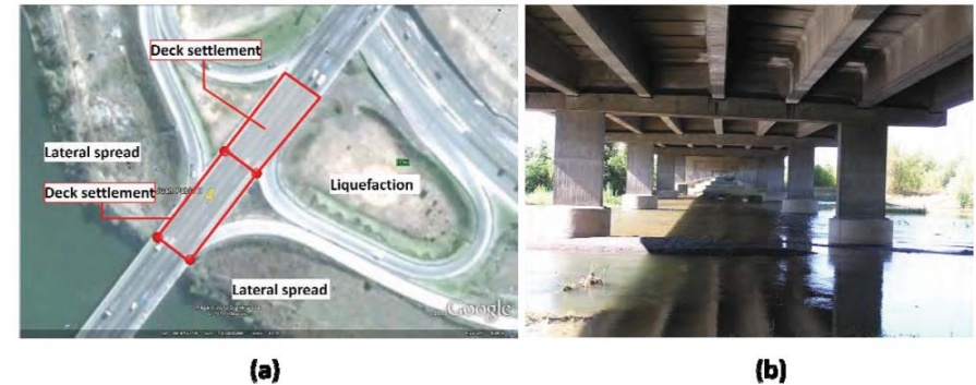
Figure 9.9. Juan Pablo II Bridge (a) Google Earth view of northeast Approach with schematics of observed damage (S36.815864° W73.083674°) (b) Typical bridge bent configuration (S36.828181° W73.095850°; 1636 hrs on 3/15/2010)
