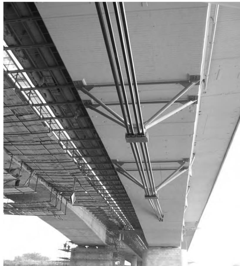
Figure 5: View of external tendons (Děčín)
