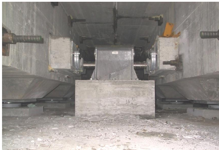
Figure 17: MELOTP Damping System as installed in a SS 147 viaduct.
