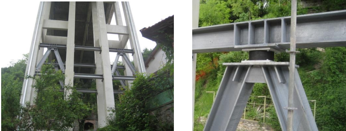
Figure 21: Chevron braces at Pier 1 (left), HDRB as installed on a chevron brace top (right)
