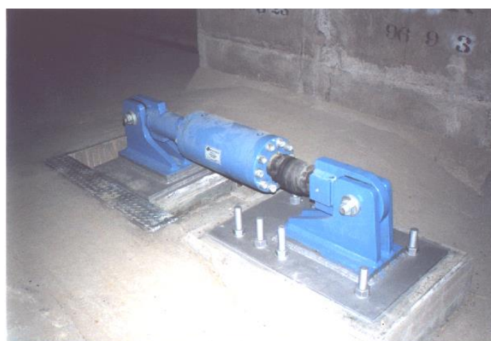
Figure 13: Viscous Damper as installed inside the box girder of the Seo-Hae Bridge Approaches.
