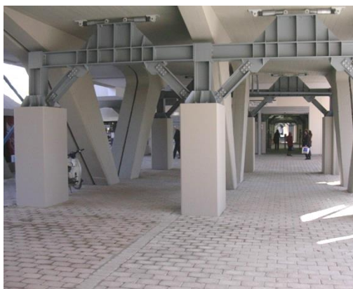
Figure 8: Isap Bridge Viscous Dampers as Installed
