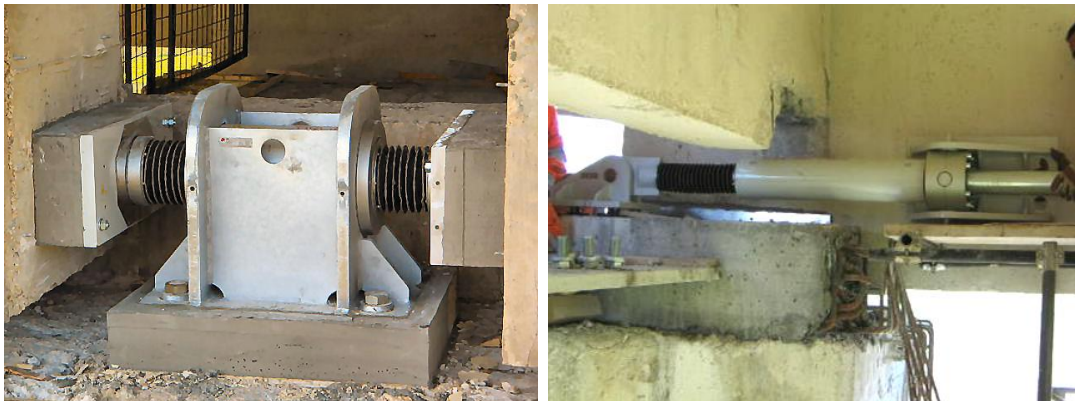
Figure 11: Carboj Viaduct: Viscous Dampers as installed in a standard pier (left) and under installation in an expansion joint pier.
