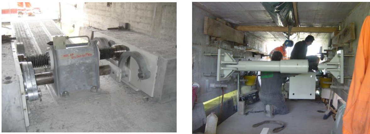
Figure 22: MELOP Damping System as installed (left), Shock Transmission connecting the decks during installation (right)
