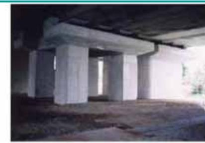
Fig. 10. 48 Seismic Retrofit using Seismic Isolation; (a) Installation of lead rubber bearings and sliding bearings, and (b) after retrofitted
