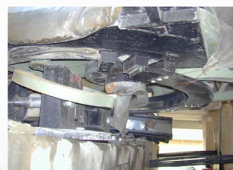
Energy Dissipation Unit (EDU) Cable restrainers
