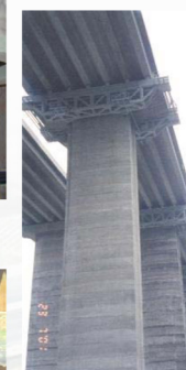
Temporary truss supports
