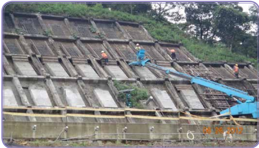
Bid No. B14 –New build ground anchors on original grid type slope protection for main line southbound
