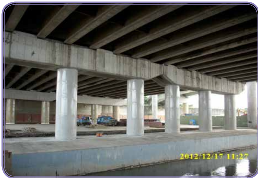
Ongoing Bid No. M12 - Tanshui River Bridge - P4 Pier column steel plate coated by II waterproofing treatment
