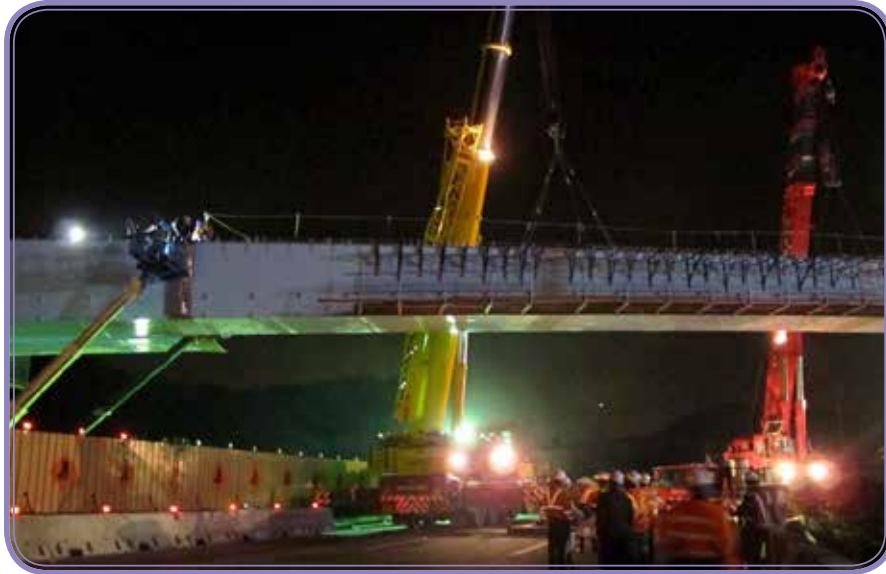
Night Lifting for Steel-box girders crossing the National No. 1 Freeway
