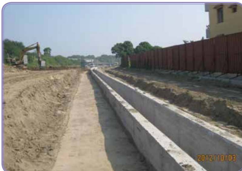
Liouying Interchange Projects - Completion of the drain ditch structure backfill construction
