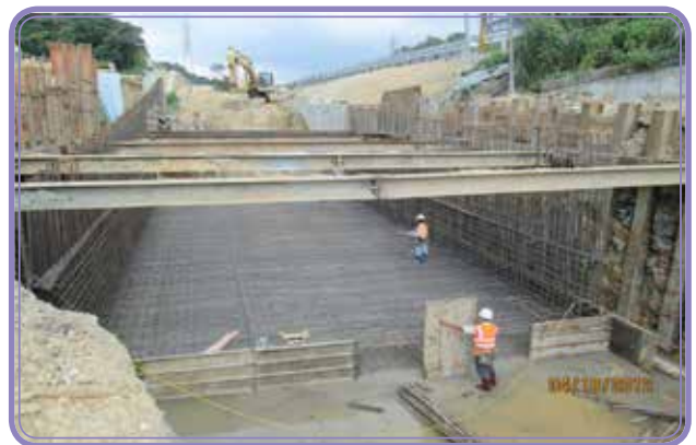
Bid No. B14 – U type retaining wall construction of Ramp R1
