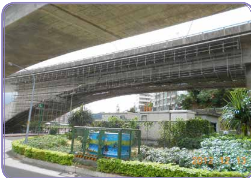
Bid No. M31 - Scaffold assembly of Bitan Bridge 5S~6S
