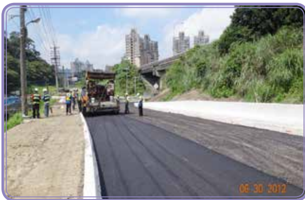
Bid No. B14 - Bituminous Treated Base (BTB) of Ramp L4 – Bid No. 14
