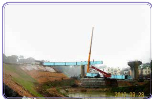
Steel-box girders lifting of P6-A3
