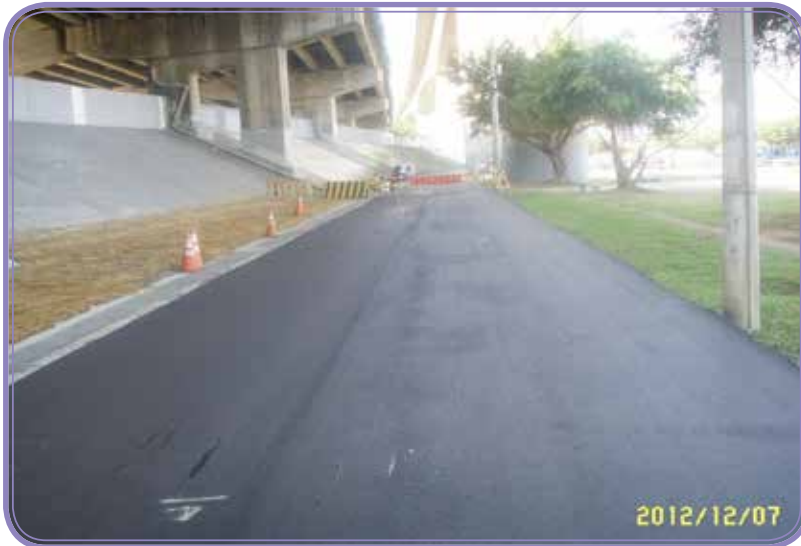
Ongoing Bid No. M12 - Yuanshan south ferry bridge – AC treated base of bike lane near the river side and P6~P7 flood prevention road
