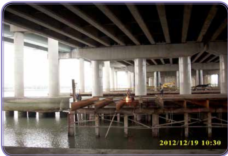
Ongoing Bid No. M12 - Tanshui River Bridge) - working platform demolition of P7 construction
