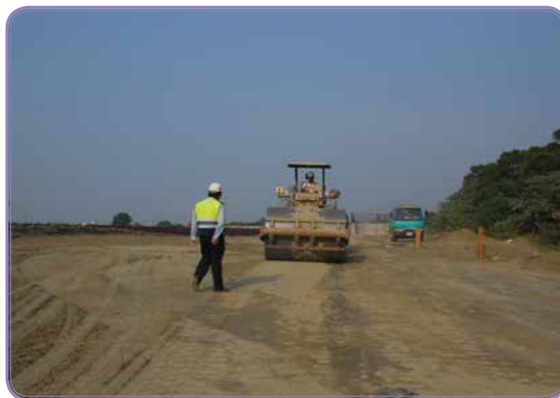
Liouying Interchange Projects - Construction situation of Embankment filling for ramp 1
