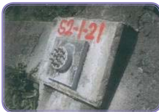
(b) Inspection on the anchor head components
