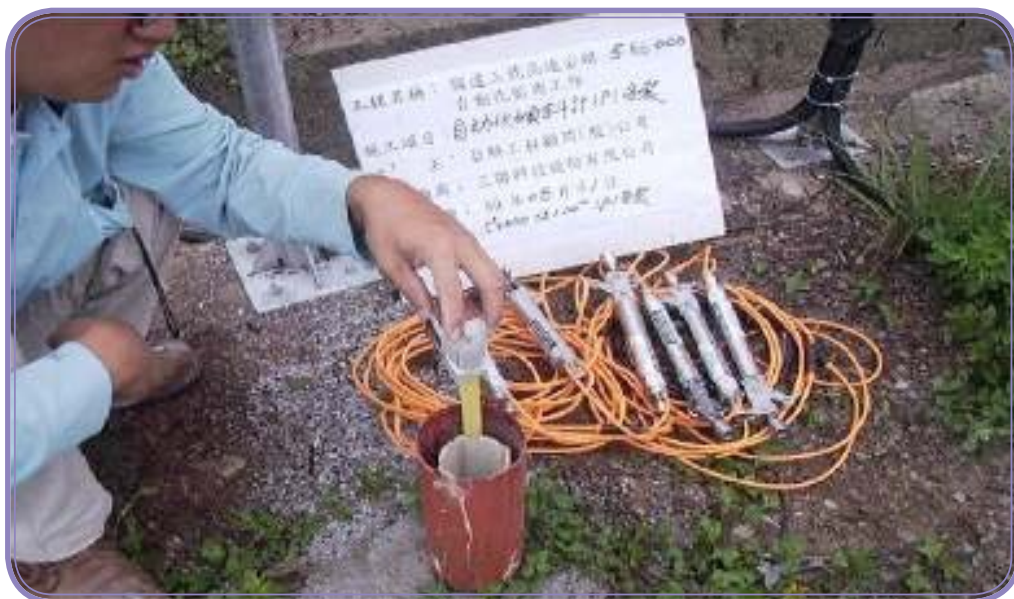
Fig. 2: Installation of automated and self-recording inclinometer.
