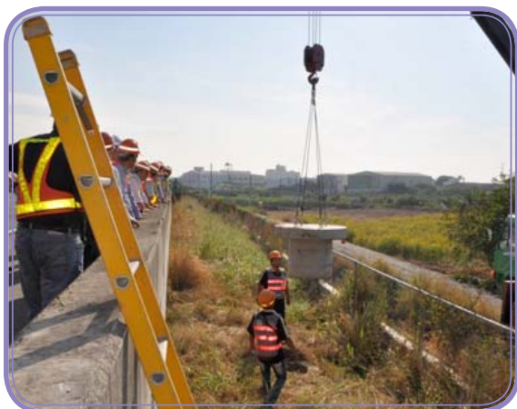
Construction works for 2-ton RC manhole covers
