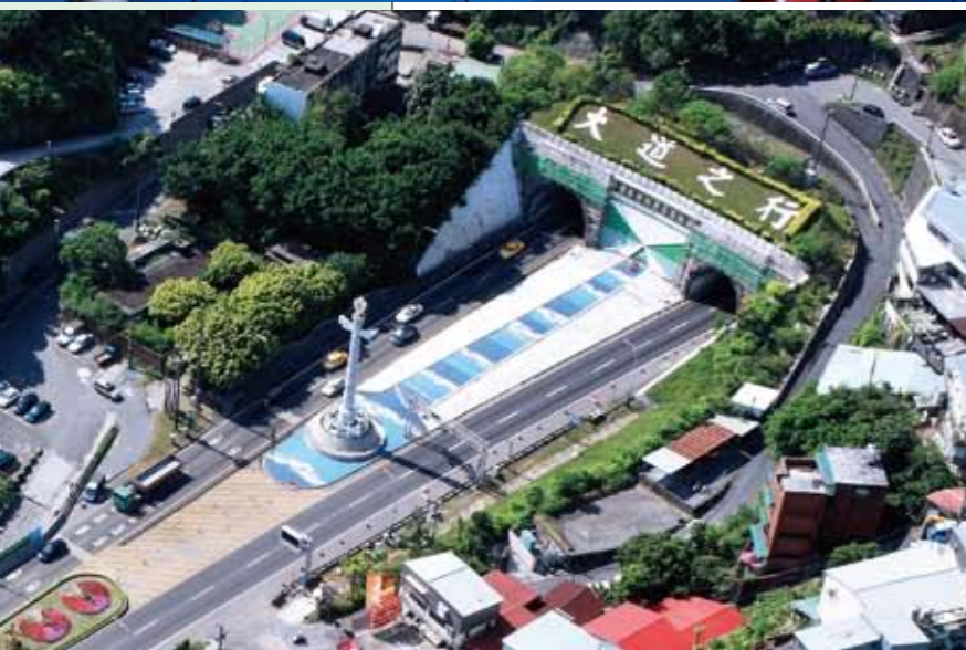
國道1號起點——基隆端。 The starting place of National Freeway No. 1 at Keelung.
