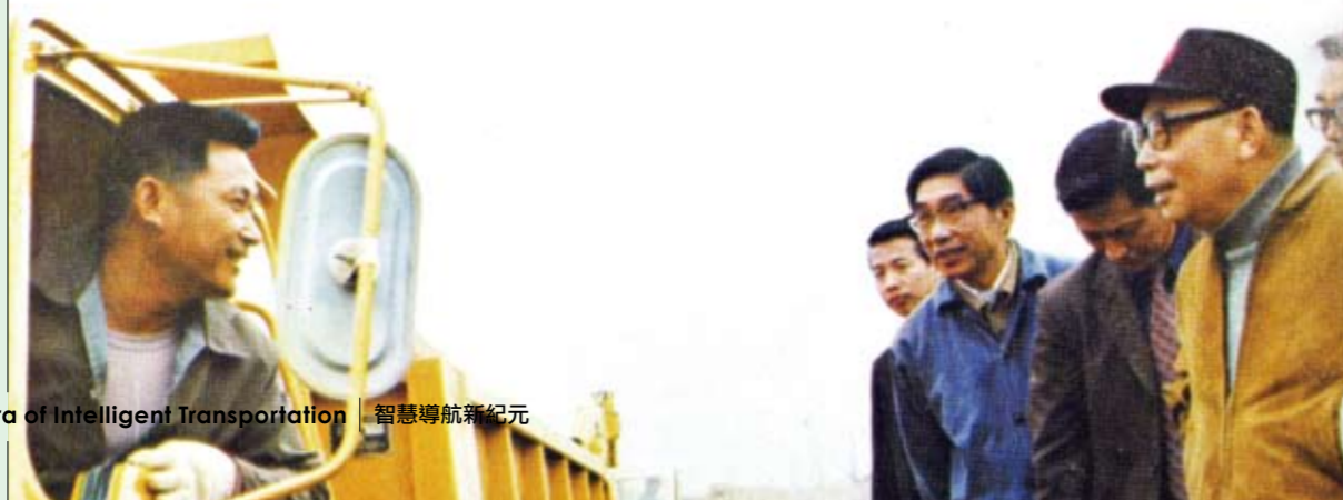
當年的行政院長蔣經國先生前往施工處視察。 Mr. Chiang Ching-kuo, the Premier of Excution Yuan at that time, inspected construction work.
