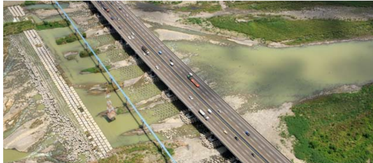
國道1號／頭前溪橋 Touchian Stream Bridge on National Freeway No. 1
