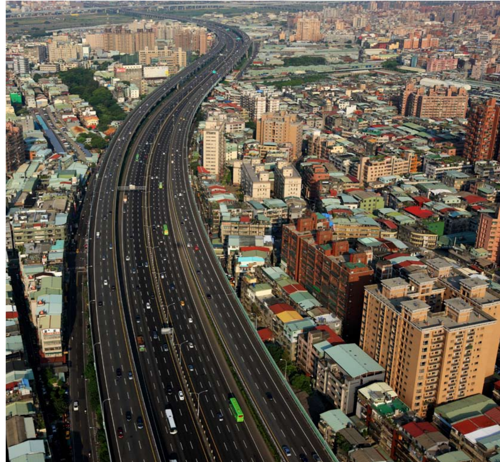
Sanchung-Wugu section of National Freeway No. 1
