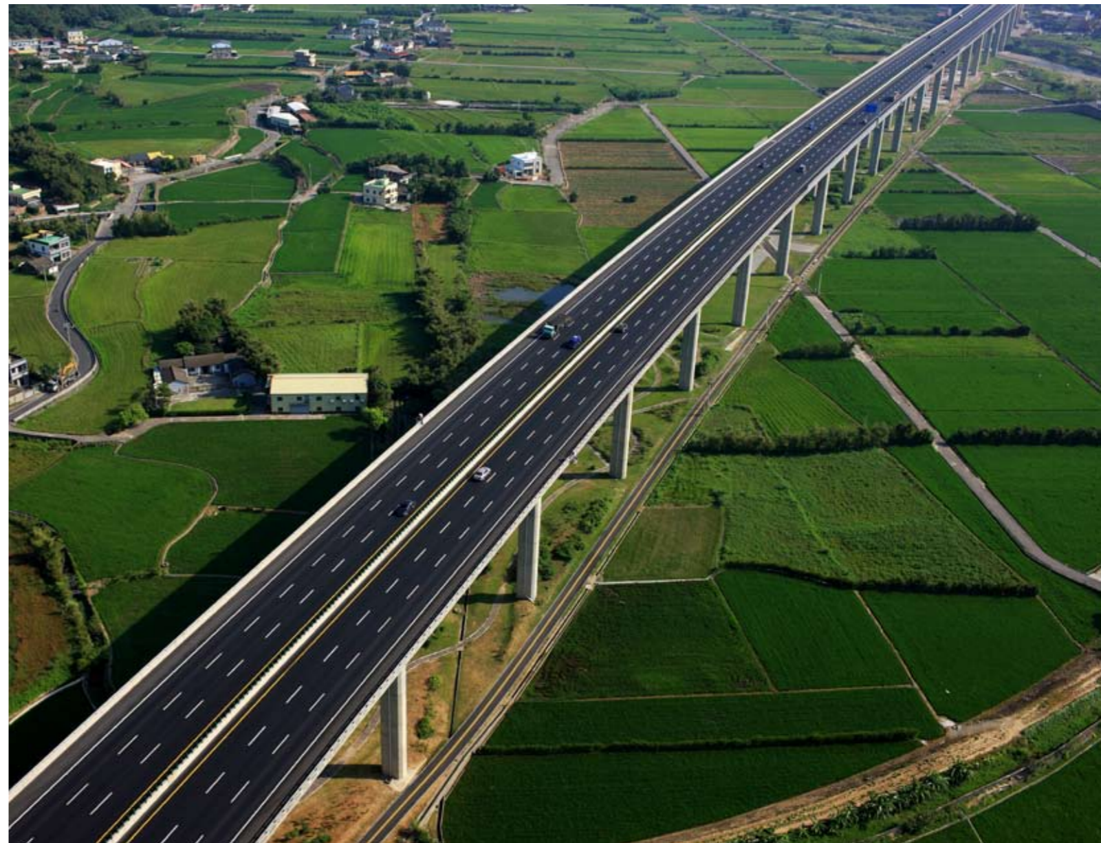
Xihu viaduct section of National Freeway No. 3
