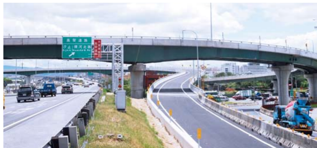
Wugu Interchange in reconstruction.
