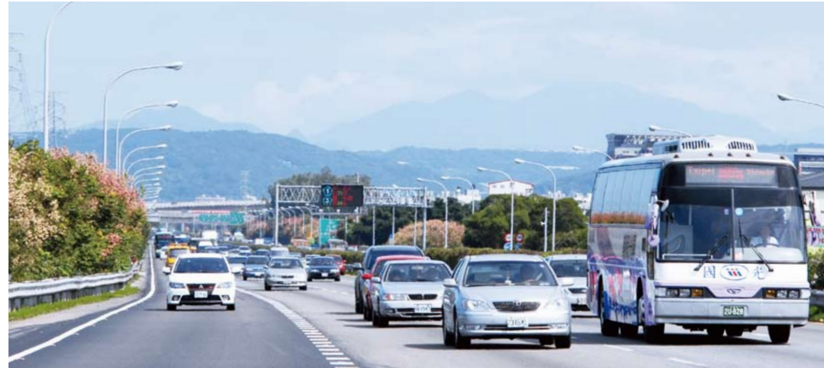
輔助車道 (國道1號/機場系統-中壢服務區路段) Setting up an auxiliary lane (Airport System to Zhongli Service Section of National Freeway No. 1)
