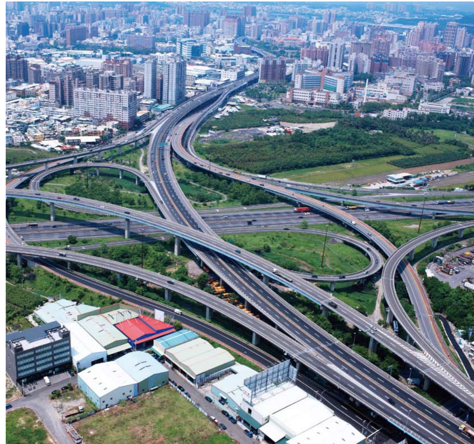
Dingjin System Interchange of National Freeway No. 1
