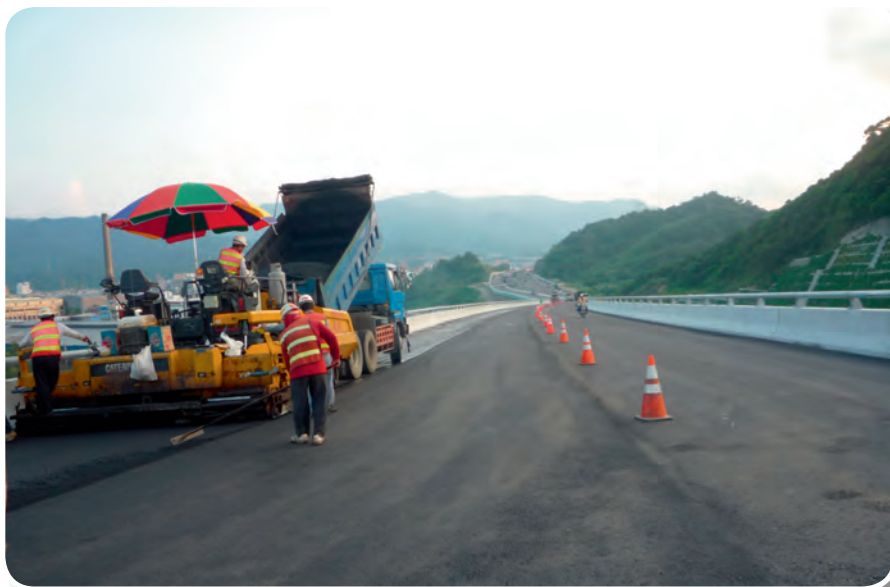
E匝道橋面AC鋪築
