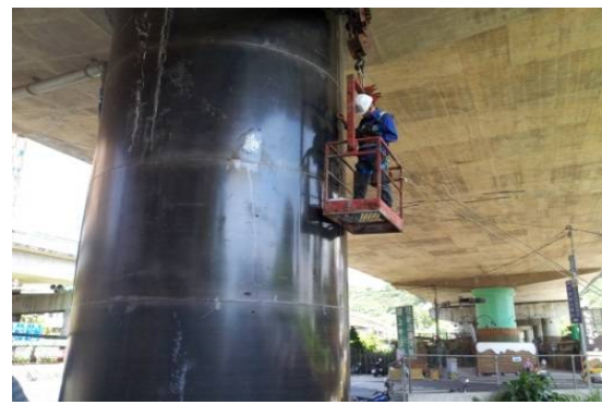
Figure 16: Steel jacketing and welding inspection
