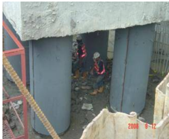
Figure 22: Steel jacking on scoured piles
