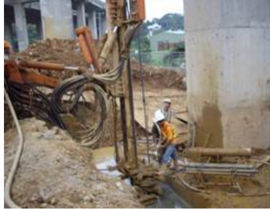
Figure 24: Micropile construction
