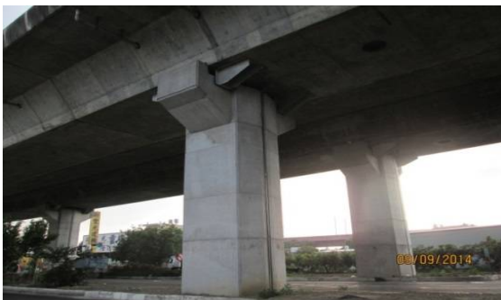
Figure 11: RC and steel aseismic device
