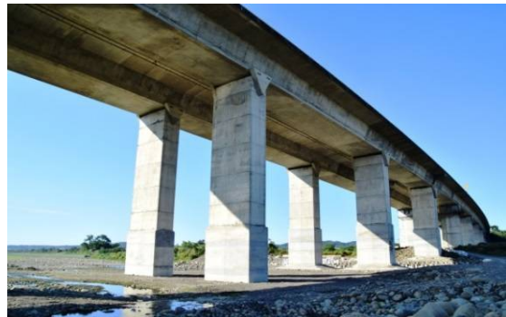
Figure 10: RC jacketing and aseismic block
