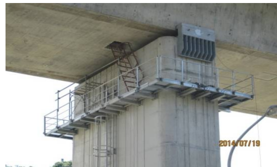
Figure 12: Transverse steel aseismic device
