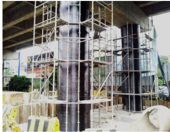
Figure 18: Column confined by a composite fiber/epoxy jacking
