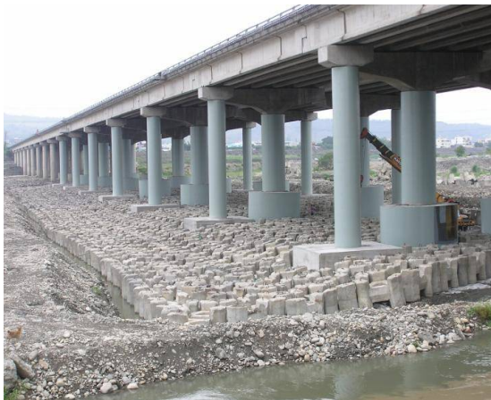
Figure 21: Pier steel jacking and scour protection
