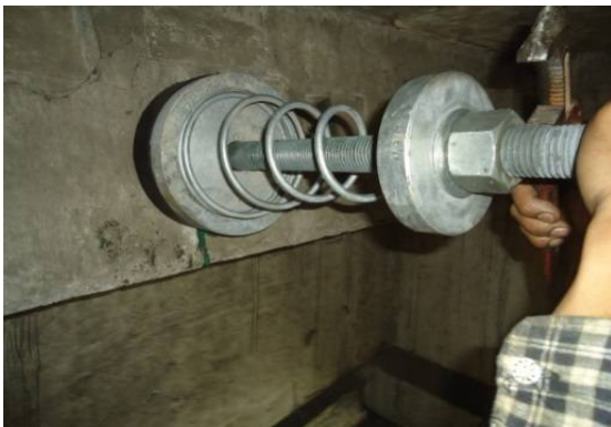
Figure 13: Longitudinal joint restrainers
