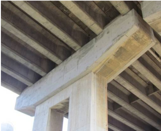
Figure 19: Strengthening of pier cap and shear keys
