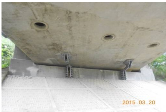
Figure 15: FVDs and shear keys
