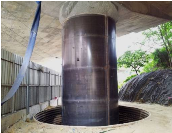
Figure 17: Steel jacking and corrugated metal excavation
