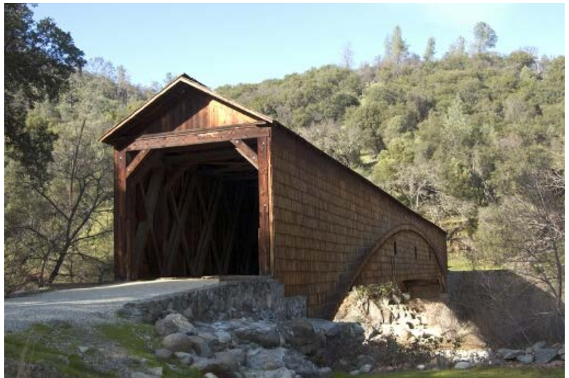
Bridgeport Bridge, Nevada County, Caltrans
