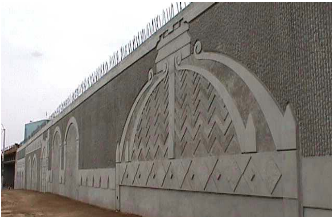
Retaining Wall, Caltrans
