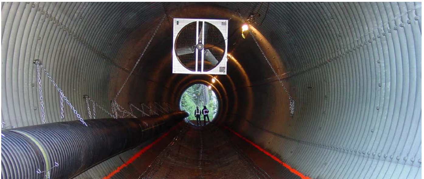
Culvert Invert Repair, Caltrans
