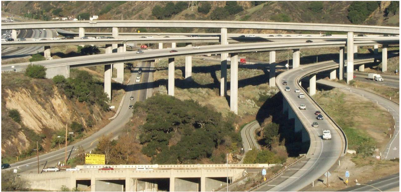
5/14 Interchange in LA County, Caltrans
