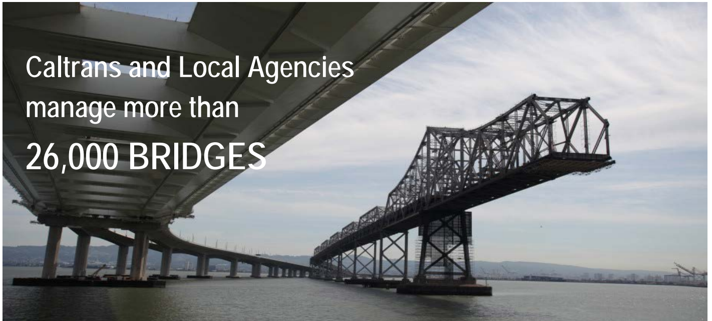
San Francisco-Oakland Bay Bridge East Spans, Hwy 80, Caltrans
