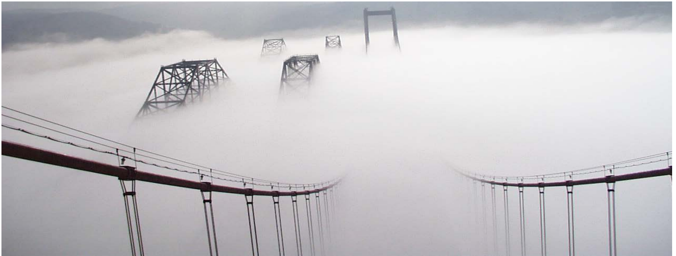
Carquinez Bridge, Hwy 80, Solano County, Caltrans
