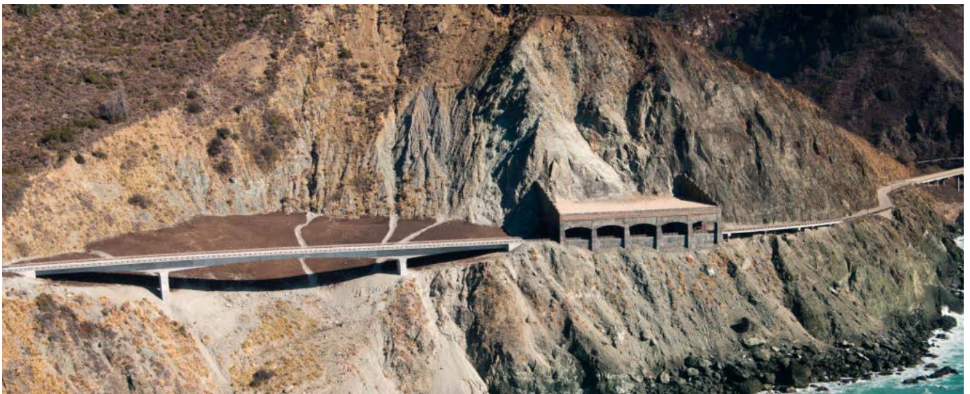
Pitkins Curve Bridge and Rockshed, Hwy 1, Monterey County, Caltrans
