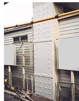
Figure 5. New seismic retrofit measures for columns [JR East , 2014]
