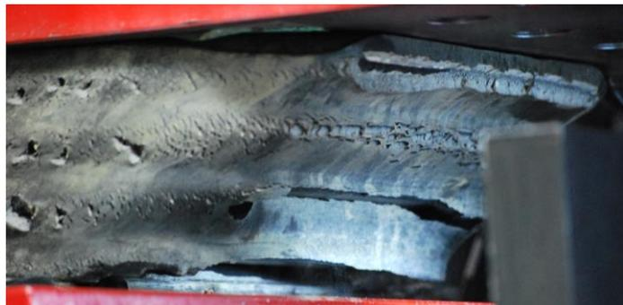
Figure 13. Ozone damaged elastomeric bearing
