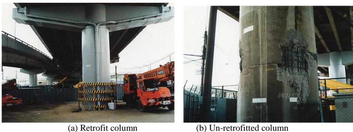
Figure 1. Effectiveness of the seismic retrofit of bridges (The case of 1995 Kobe earthquake) (Tsukimiyama viaduct, Hanshin expressway) [ADACHI et al, An analytical study of damaged viaducts due to the Great Hanshin Earthquake using estimated input ground motion, 1997]
