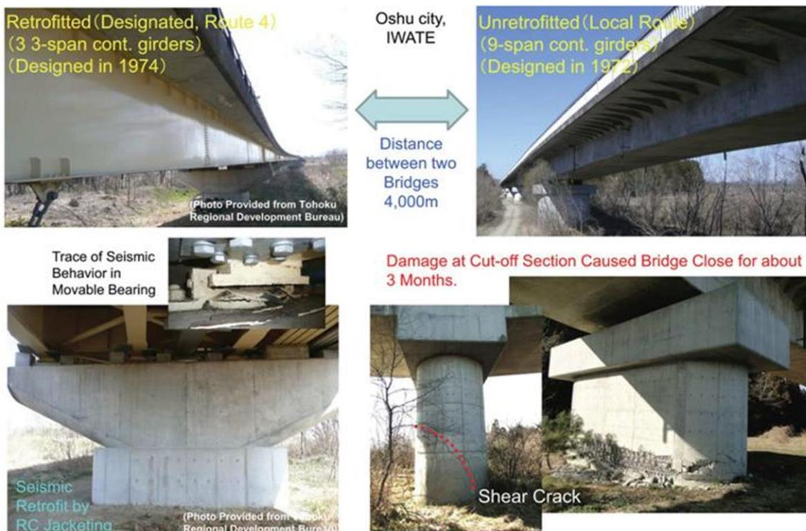
Figure 2. Effectiveness of the seismic retrofit of bridges (The case of 2011 East Japan earthquake)
