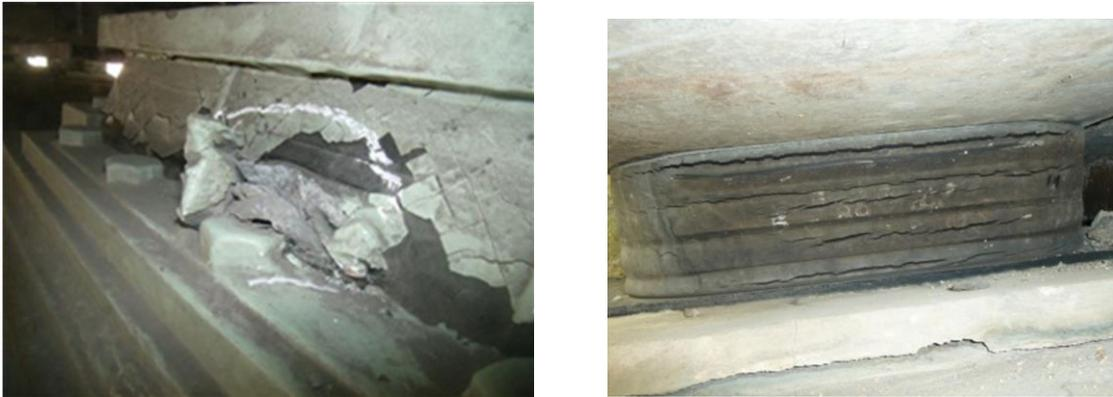
(a) Lead leaking out (LRB 17 years in-service) (b) Ozone crack (RB 27 years in-service)
