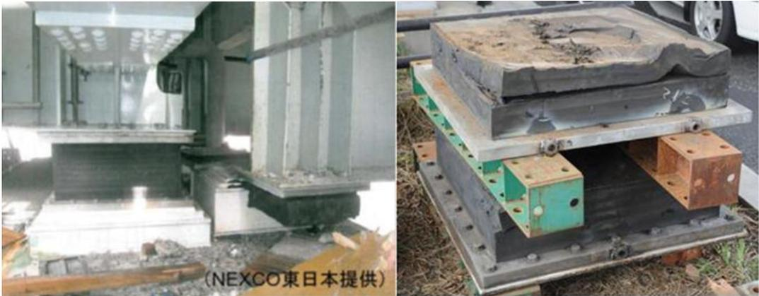
(a) Dislocation of girders due to RB damage (b) Close view of damaged RB
