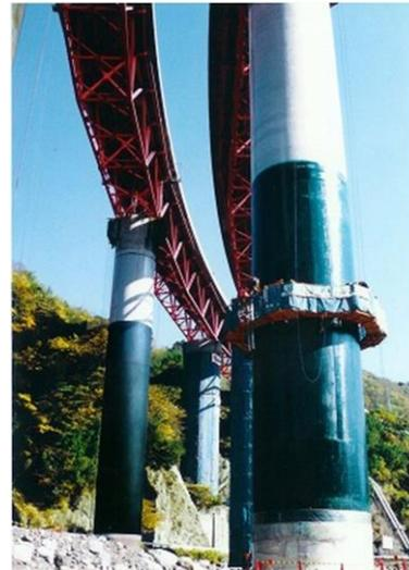
Figure 4. Carbon fiber jacketing method [OSADA et al, 2000]
