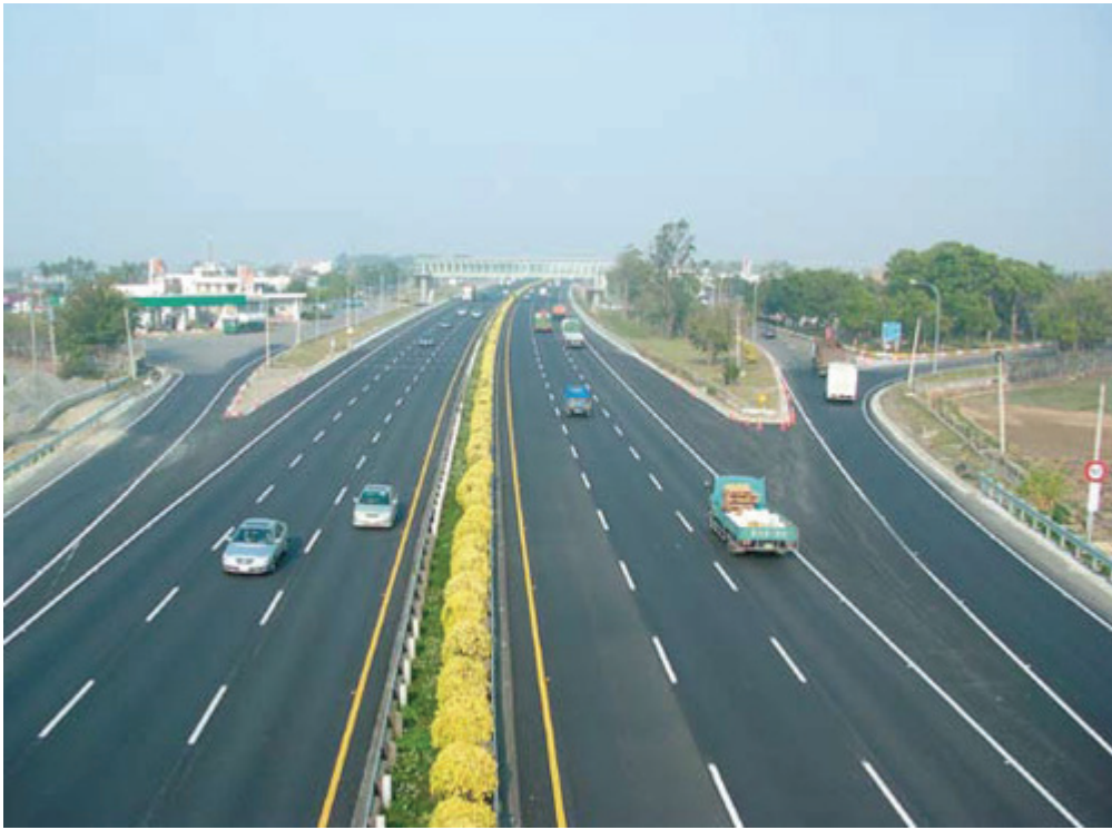
Project No. 541—completed the widening on Jan 31, 2007
