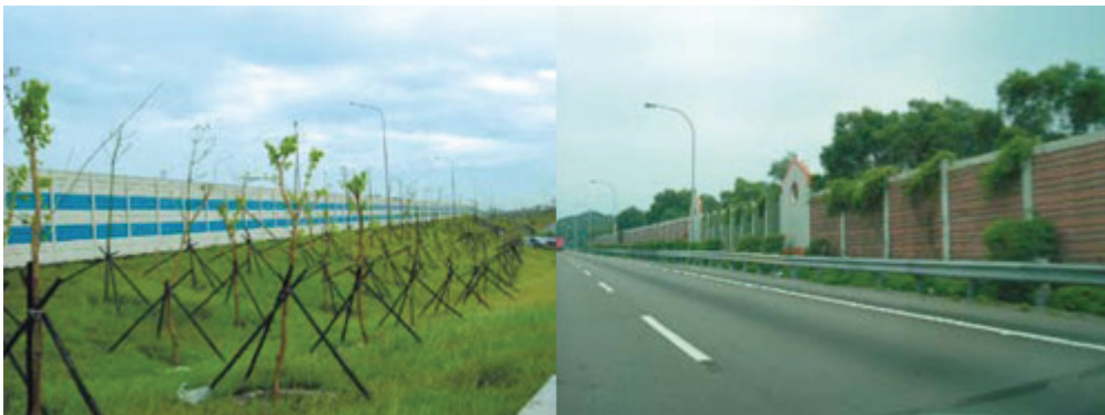
Utilising noise barrier and surrounding landscapes to enhance road scenery.
