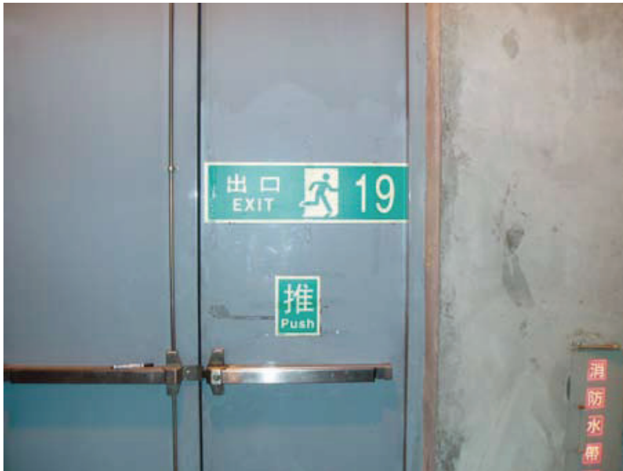
Emergency exit number and safety door opening instruction signs.
