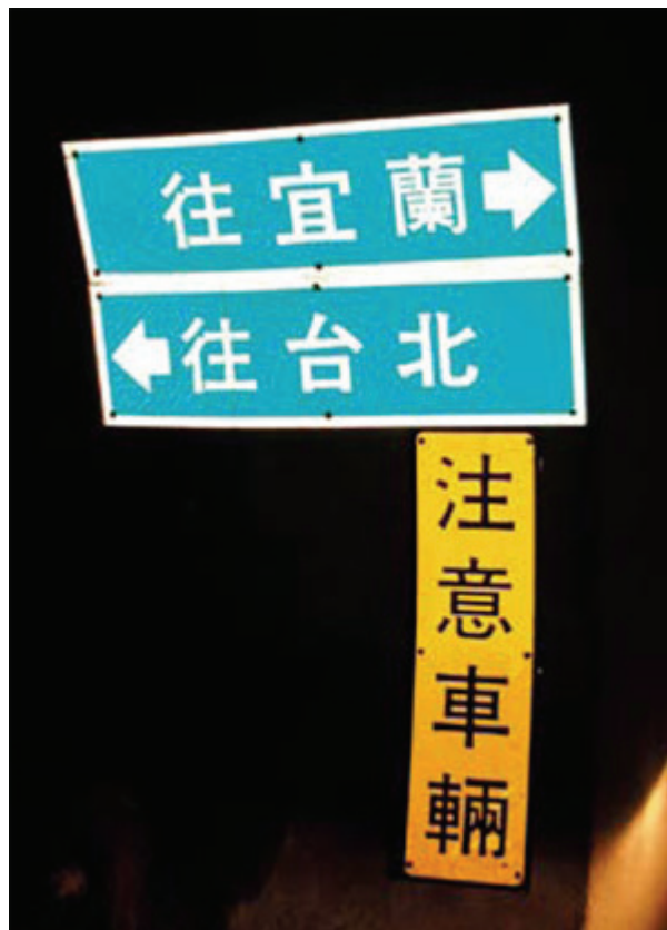
Sign installed in pilot tunnel.
