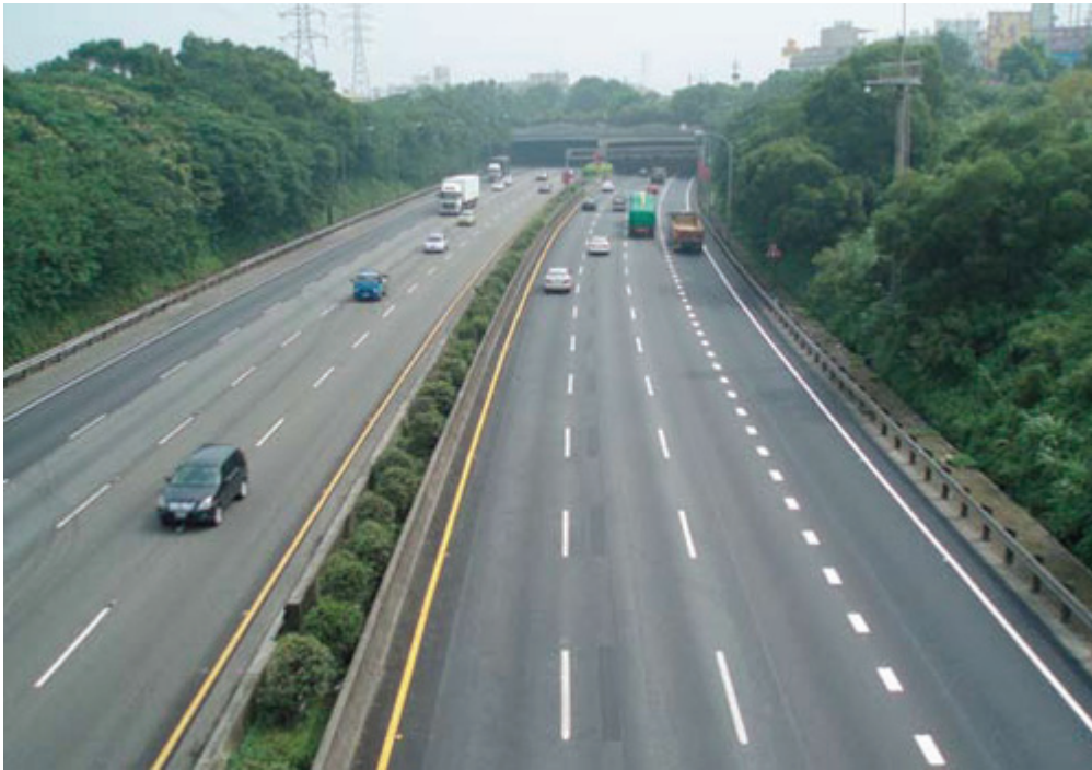
Freeway No. 3 Dasi to Puding tunnel exit northbound section with added auxiliary lanes (3 lanes to 4 lanes).
