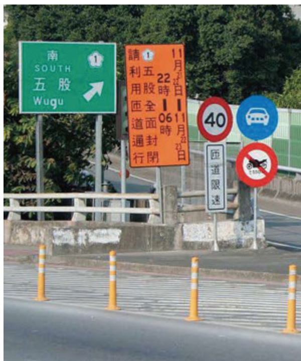
Prohibit section connecting Opened section - Freeway No. 1 Sijhih-Wugu elevated road Huanbei interchange entrance (set up Prohibitory 2.1 sign)
