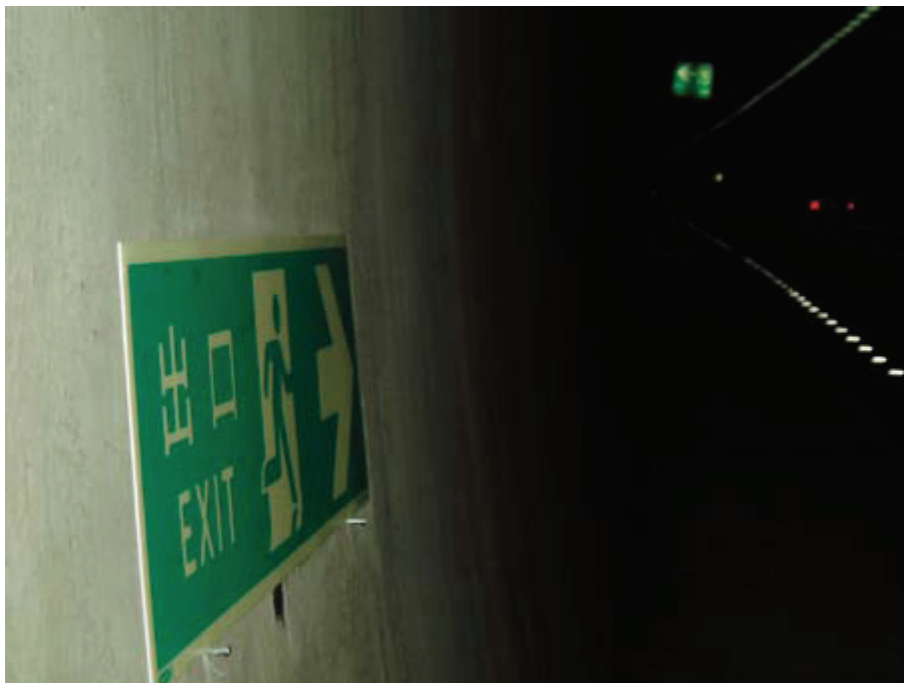
Emergency exit direction signs.
