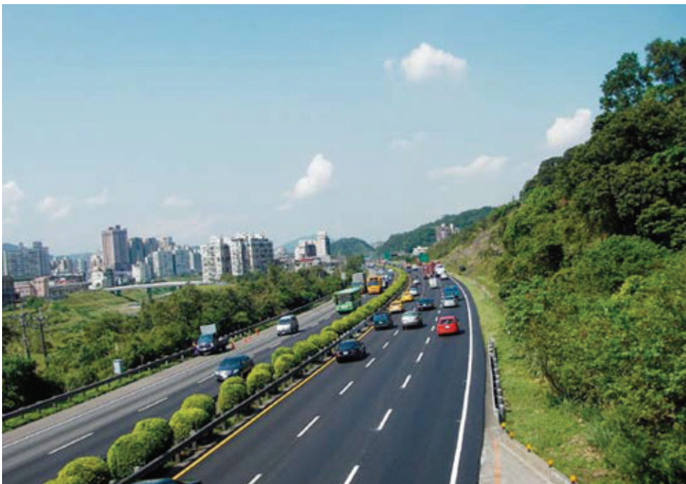
No.1 Wudu to Sijih toll station southbound section with added auxiliary lanes (2lanes to 3 lanes).
