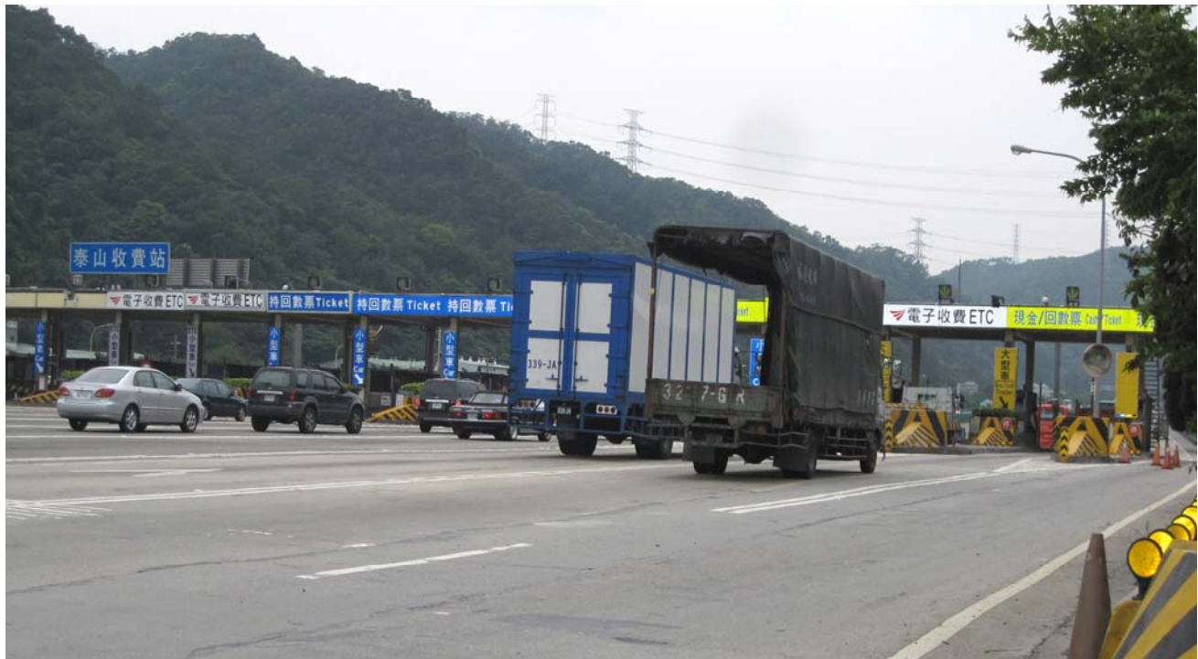
Taishan toll station ETC lane
