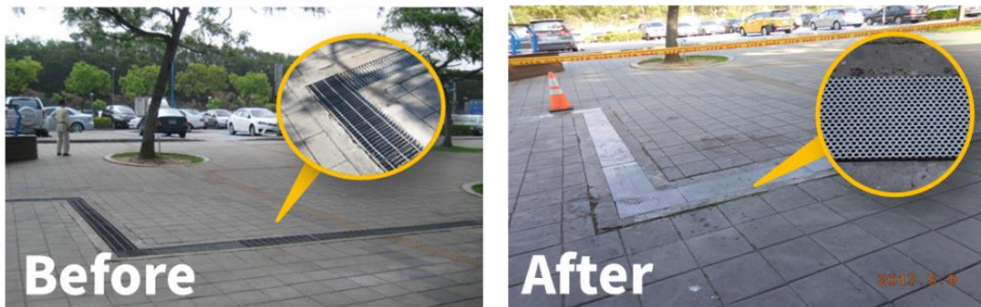
[排水溝蓋加裝細目金屬網板]
