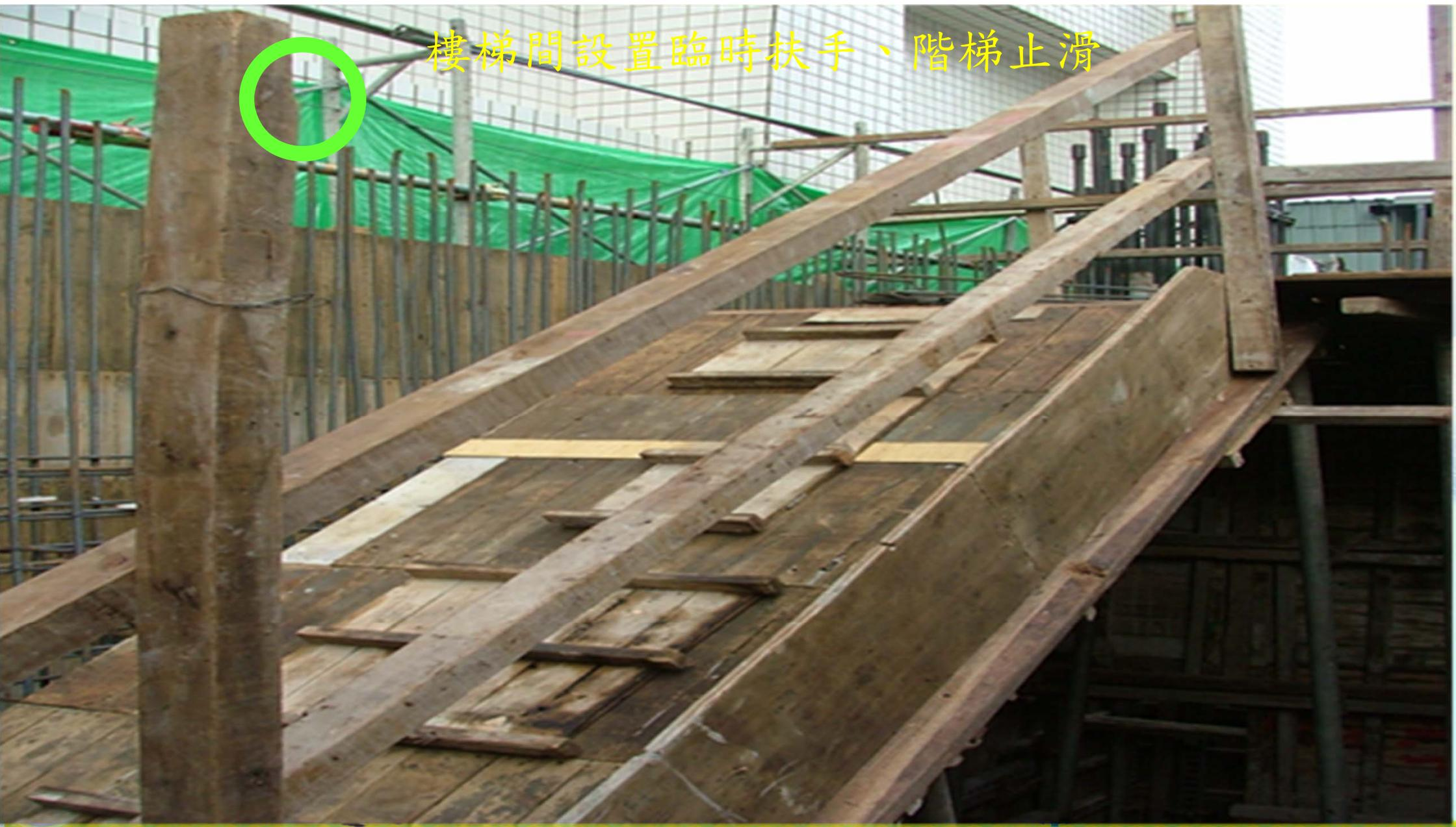
施工架與構造物間之間隙有墜落之虞
