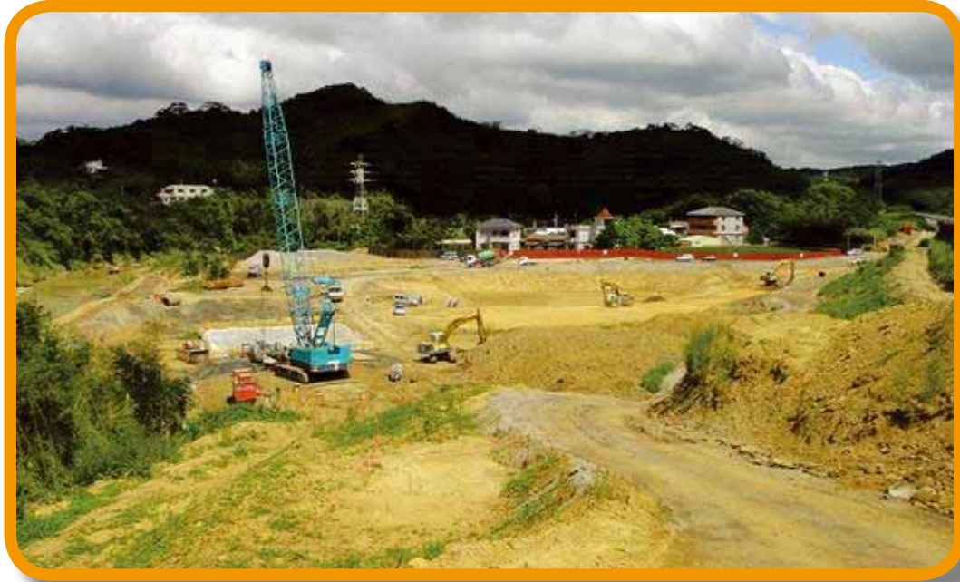
Piling and DSR1 flood detention pond works
