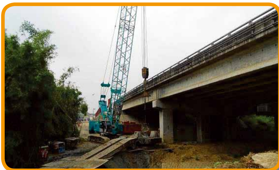
P15 full circulation piling operations
