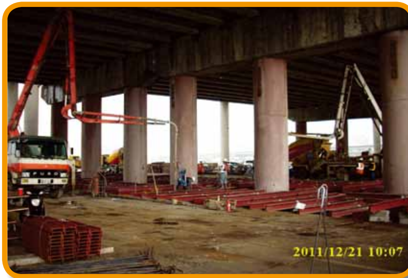
Retrofitting the piers of the bridge over the Tamshui River as ongoing bid M12 works in the bridge seismic assessment and retrofit project
