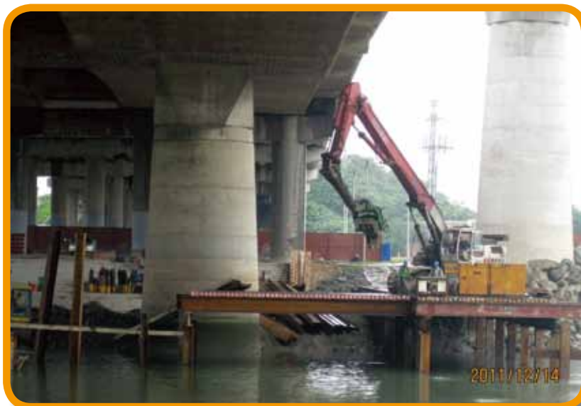
Retrofitting the piers of the bridge over the Tamshui River as ongoing bid M12 works in the bridge seismic assessment and retrofit project
