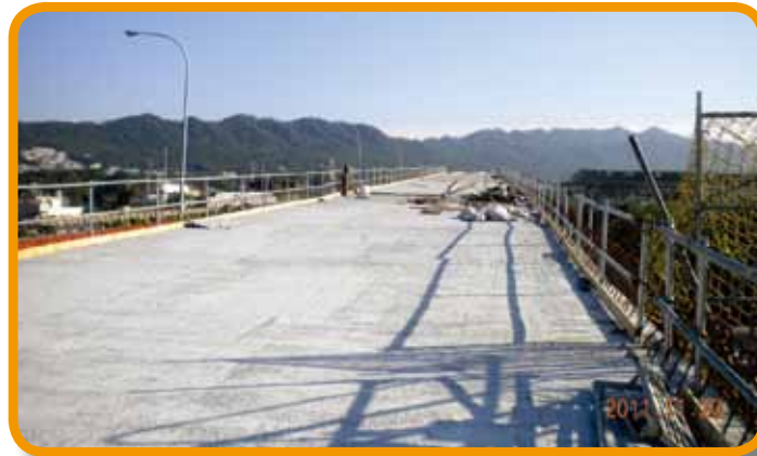
RC pouring for bridge deck AA1~PA7 in Ramp A
