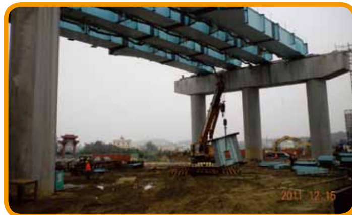
Hoisting P5~P6 steel box beams
