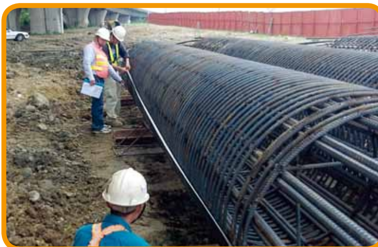
L1 ramp pile steel cage measurement examination
