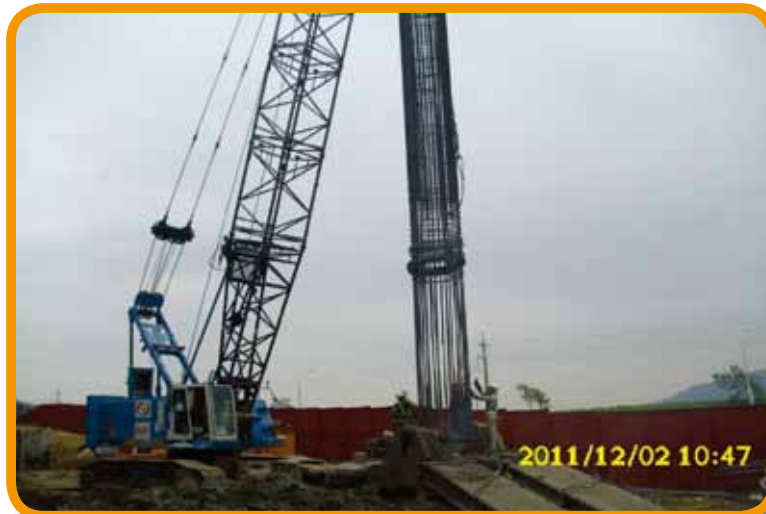
L1 ramp steel cage hoisting
