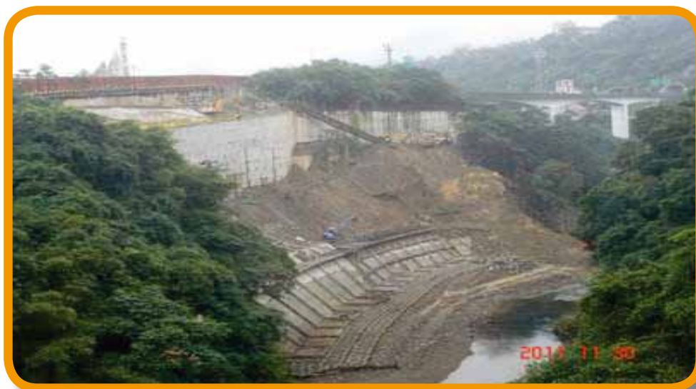
Concrete revetments, retaining walls and MRC backfilling
