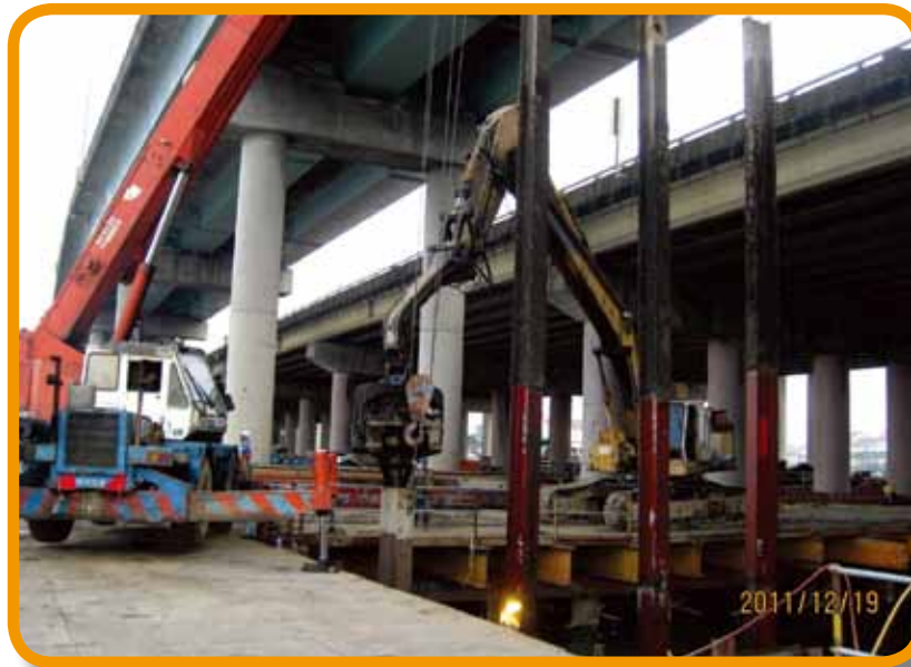
Retrofitting the piers of the bridge over the Tamshui River as ongoing bid M12 works in the bridge seismic assessment and retrofit project
