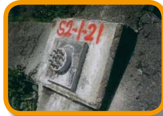
(b) Inspection on the anchor head components
